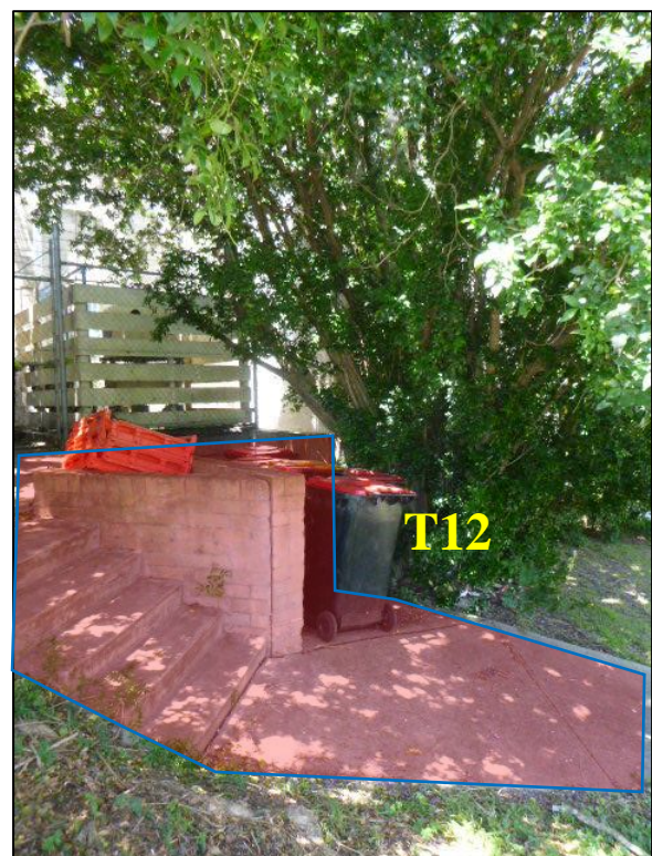
Photo 9 - Demolition of existing structures within TPZ / SRZ
