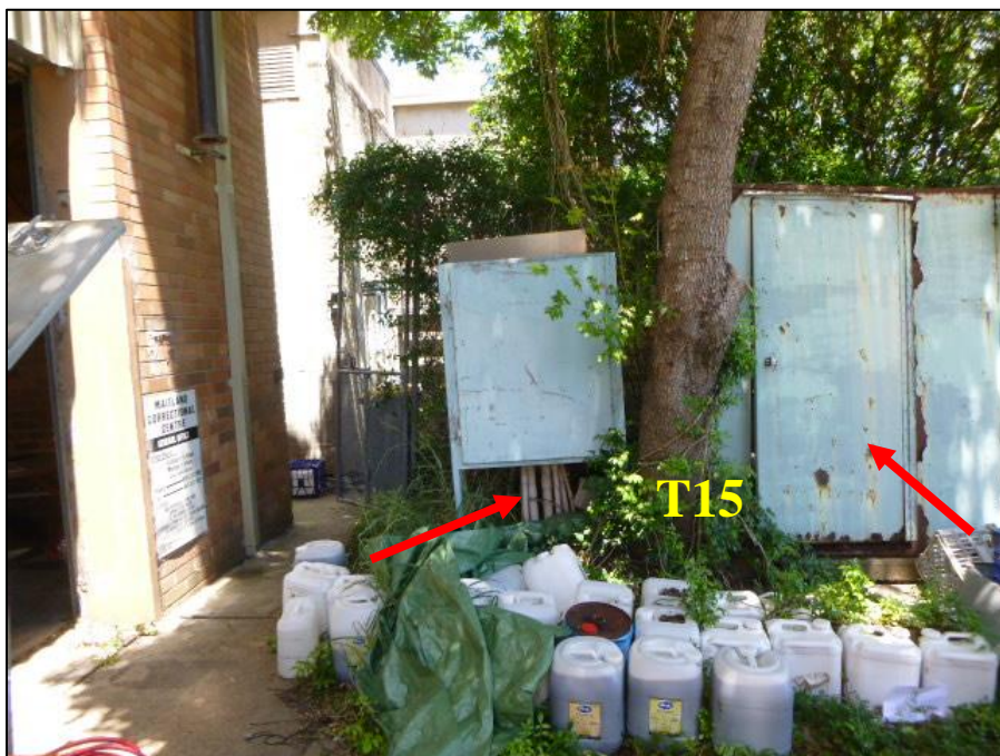
Photo 14 - Removal of generator and associated cables within SRZ
