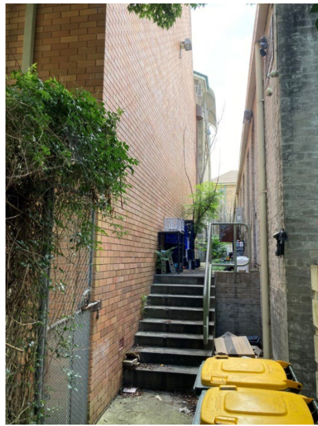
View to southeast showing rear of the café building, Gaol walls and change in levels leading up to the café terrace
