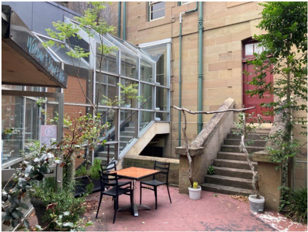
View to southeast showing former Lieutenant Governor's Residence and café terrace
