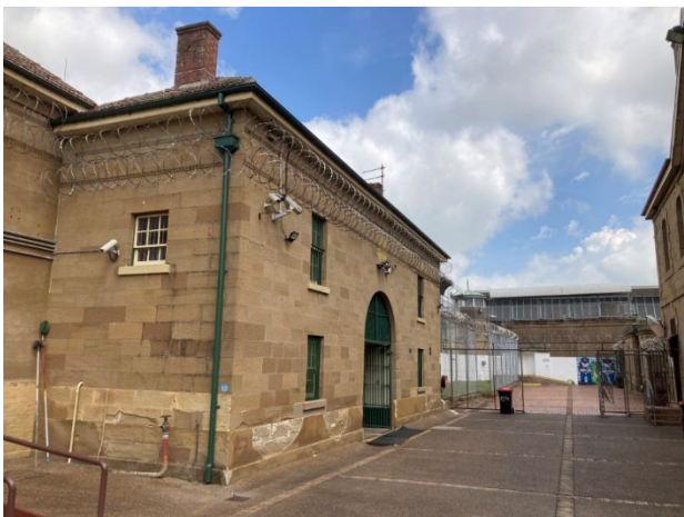
View to northwest showing gate house and internal courtyards
