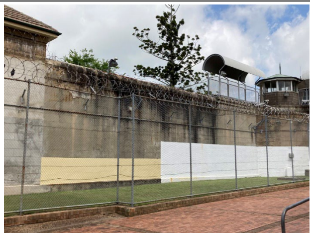
View to southwest showing Gaol wall and tower
