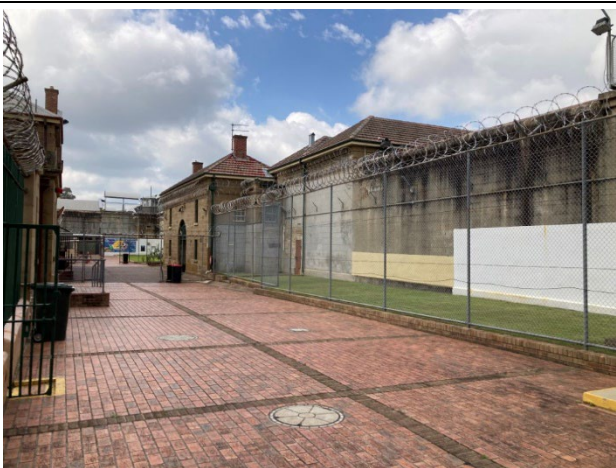
View to southeast showing internal paved courtyard
