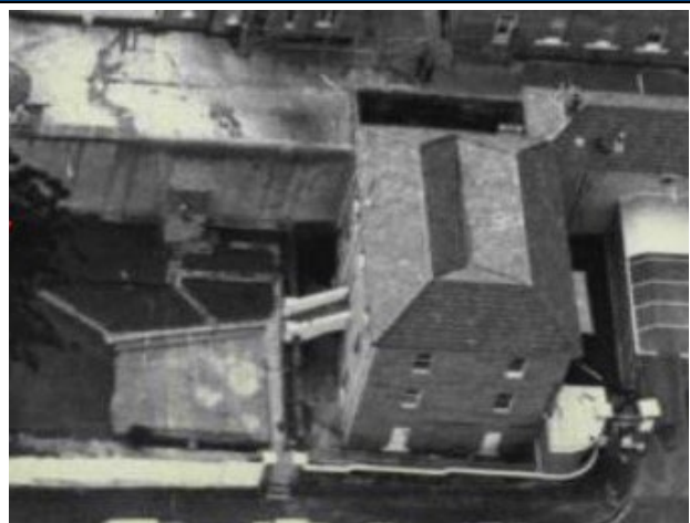
Detail of 1978 aerial showing the Warden's Quarters garden.
