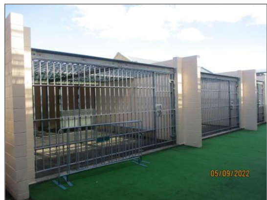
Figure 29 View of the Eastern Extension. Shows the new Yards in the foreground and the cell block behind.
