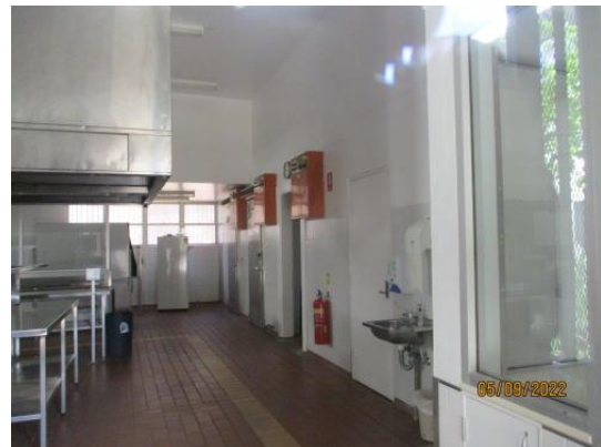
Figure 19 Kitchen Interior – Ground floor
