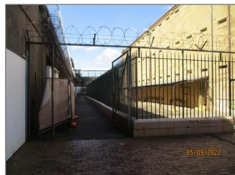
Figure 55 Typical security fences etc. (Eastern Extension)
