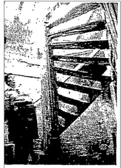
Figure 34 Interior photograph of the early timber stair inside a triangular.
