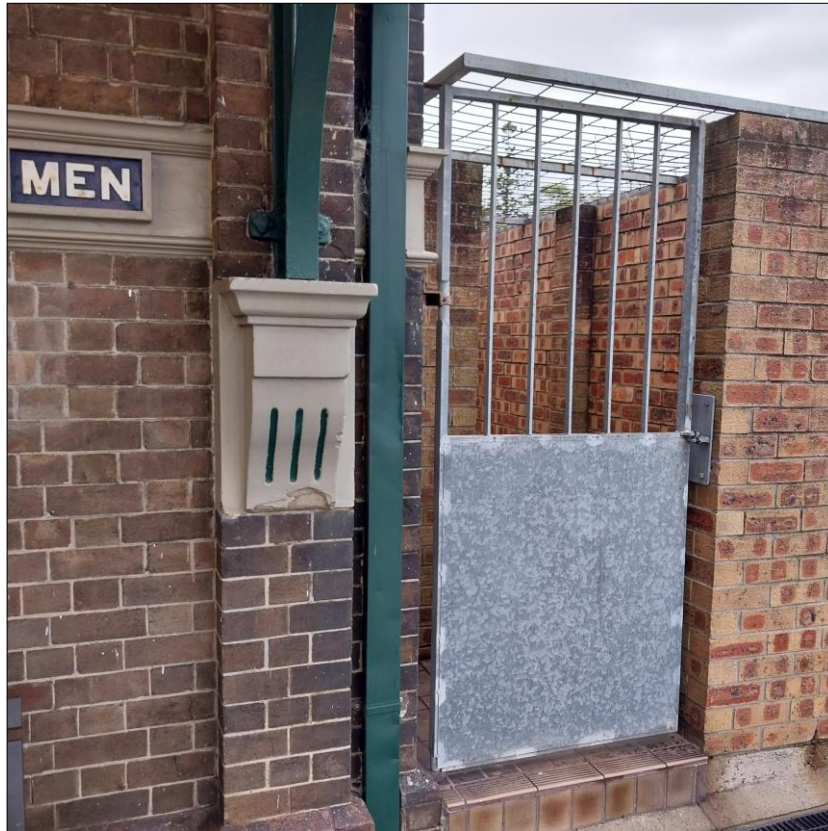
Figure 16 East Maitland Train Station Men's Bathroom. Source: Barr Planning 2023
