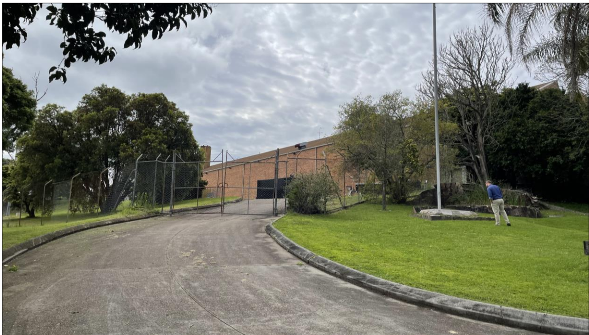
Figure 6 View of Asset Building 14 from John Street (looking southeast). Source: Barr Planning
