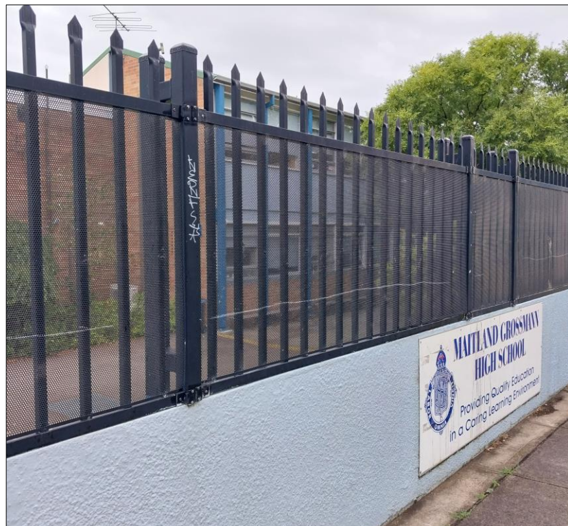
Figure 13 Maitland Grossman High School frontage. Source: Barr Planning
