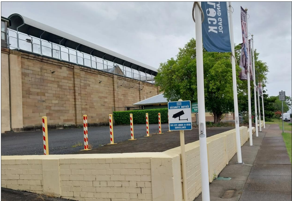
Figure 10 View of Maitland Gaol from John Street (looking north). Source: Barr Planning
