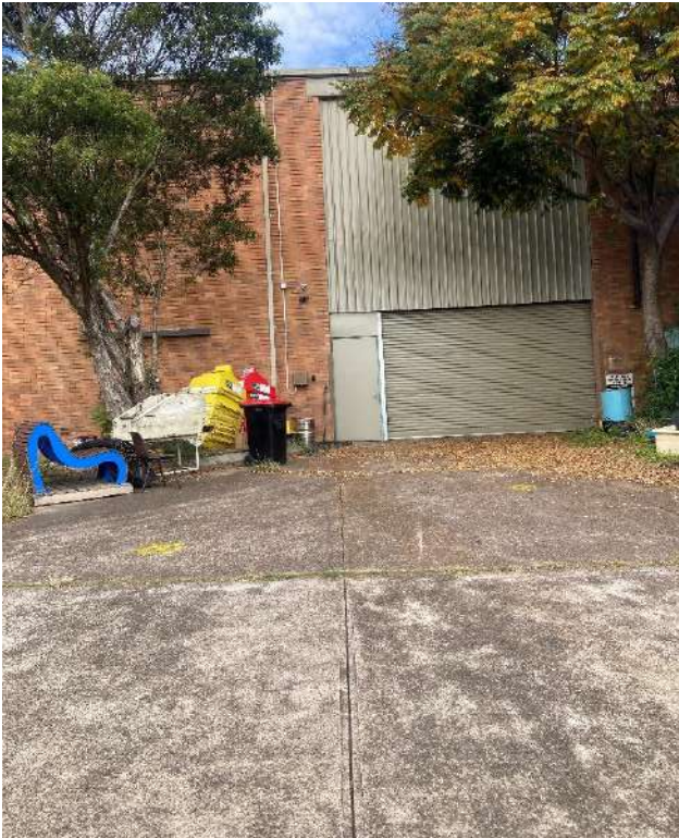
Photograph 4 – Rear roller door storage area of Gaol, storage of various items
