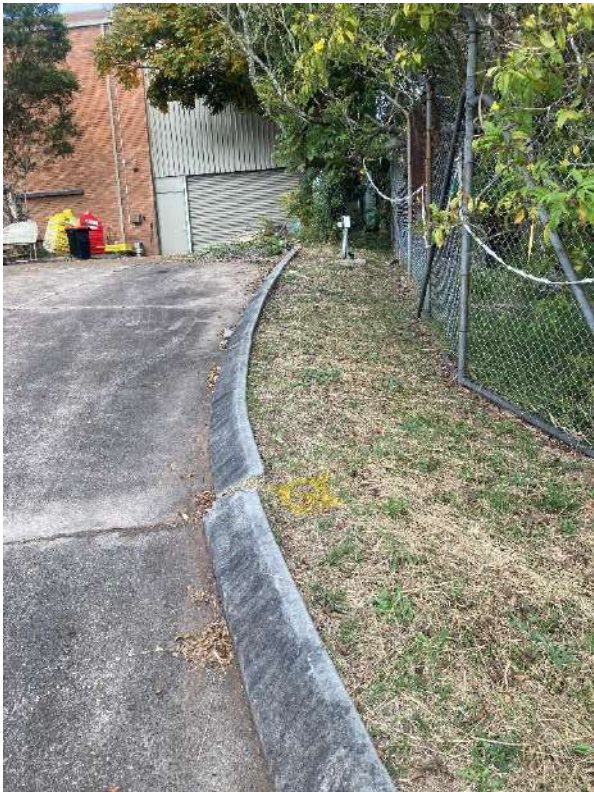
Photograph 5 – Curb of concrete hardstand driveway, cleared marking of BH7/MW3 location
