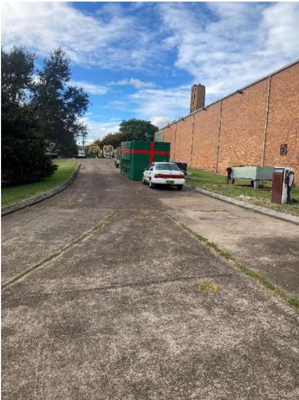
Photograph 3 – Existing concrete pavement facing Northeast
