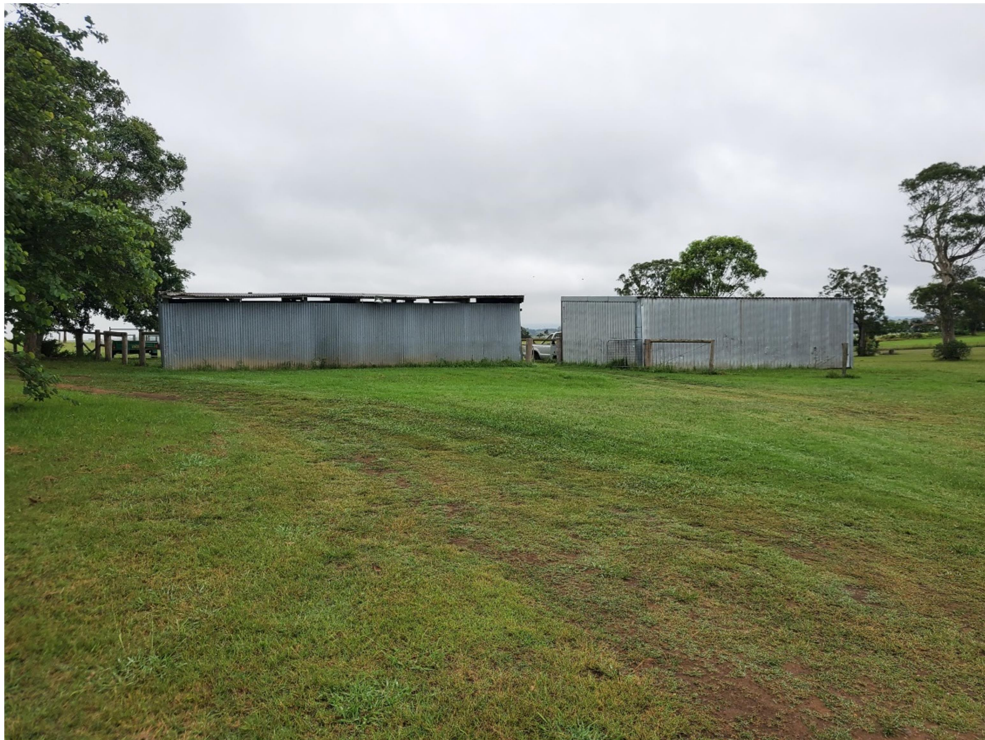
Photograph 14: View of the two sheds, facing east.
