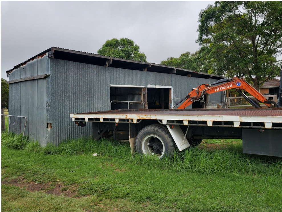
Photograph 12: Shed with truck and excavator.
