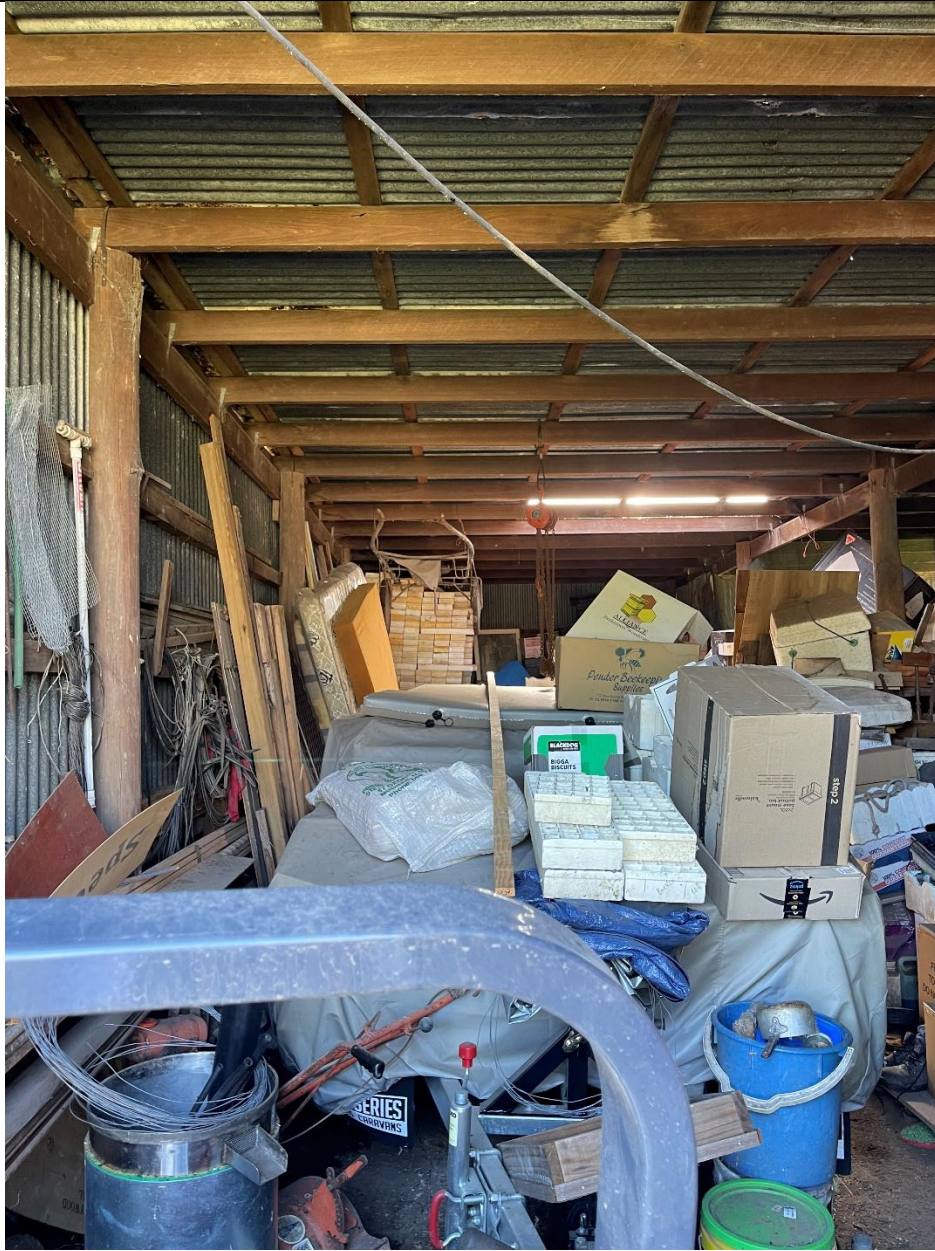
Photograph 9: View of the interior of the shed on site, looking north.
