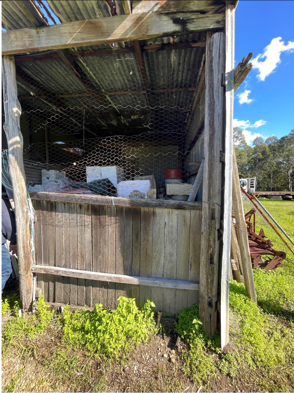
Photograph 7: View of the northern portion of the shed, contents primarily comprise beehives (no longer in use).
