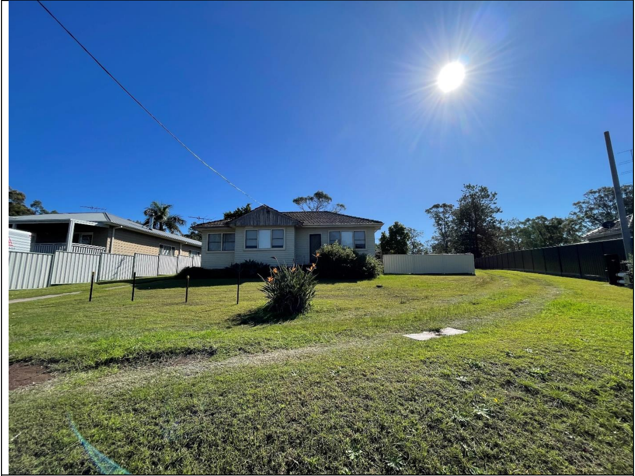
Photograph 1: View of the dwelling on site, looking north.
