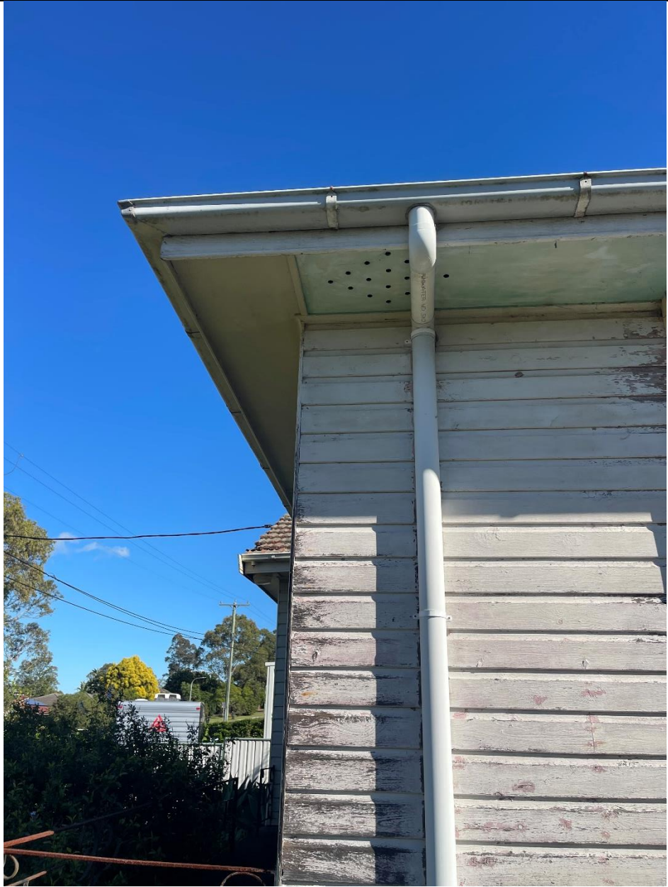
Photograph 2: View of the dwelling's eaves.
