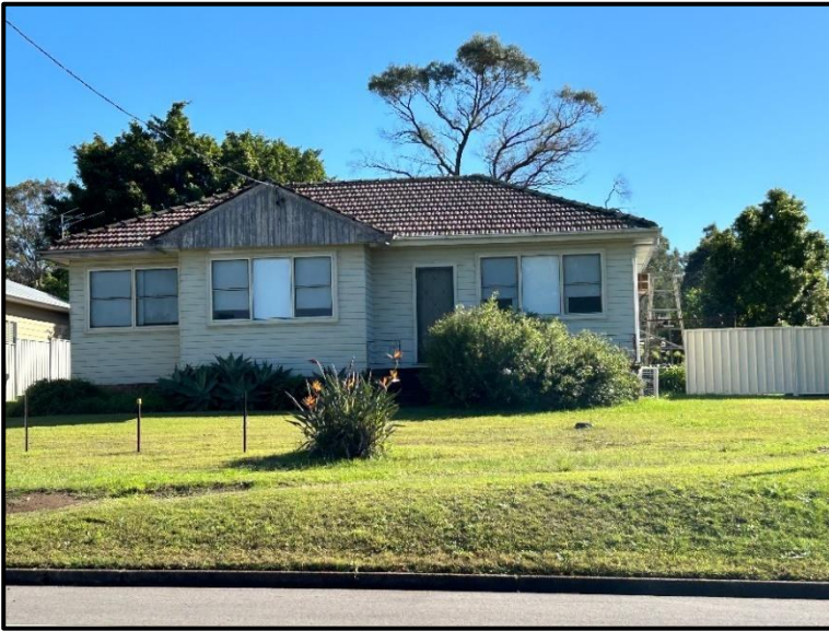
Photo 1: Subject site, as viewed from Paterson Road
