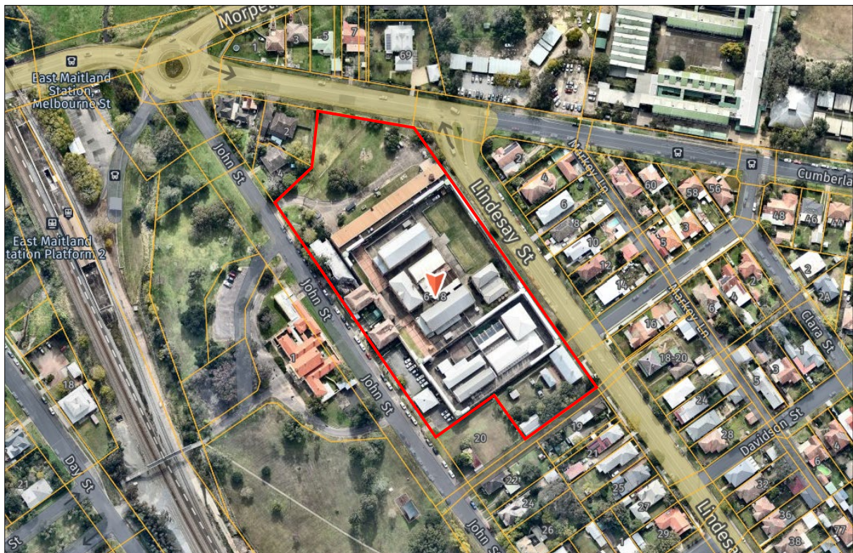
Figure 1 Site Aerial Image. Source: Near Map (August 2022)
