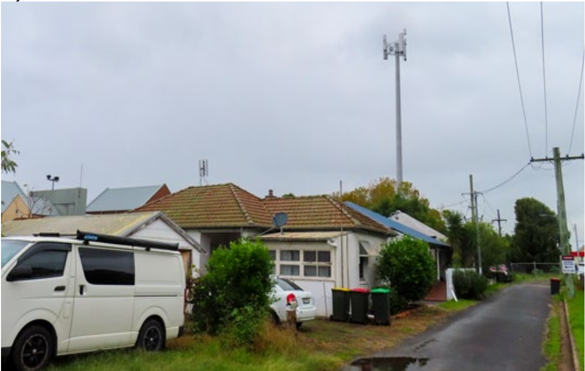
Figure 22 - Photo Montage 3: From Corner of Denman Street and Lintott Lane, looking south
