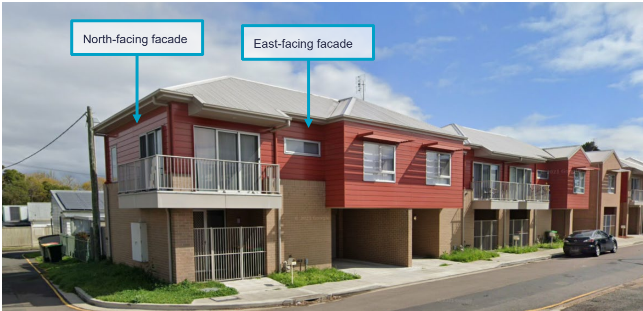
Figure 30: View of the southern-most dwelling on 6 Little Hunter Street and the only one with a façade facing the proposed facility. There is a small balcony area facing the proposed facility, but the majority of it, including sliding doors and other windows, is clearly aspected to take in views to the east, and not south towards the proposed facility. This, and the others on the same property, are the only two storey residences in the small residential pocket north of the proposed facility.
