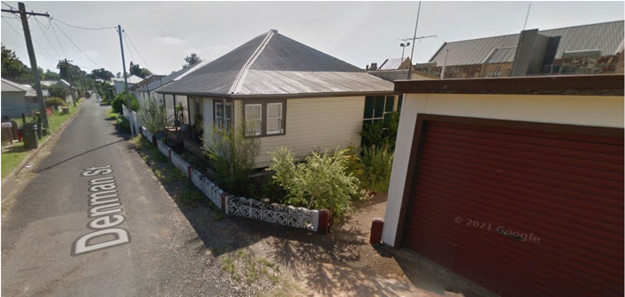
Figure 25: View of the south-facing wall of 47 Denman Street, a property adjacent to the subject site. Only two small south-facing windows are in evidence, and these look out on a small outdoor area next to the garage, which is built to the boundary (Source: Google Maps).
