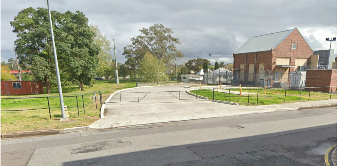
Figure 9: Existing crossover and internal access to the Ausgrid property (Source: Google Maps)
