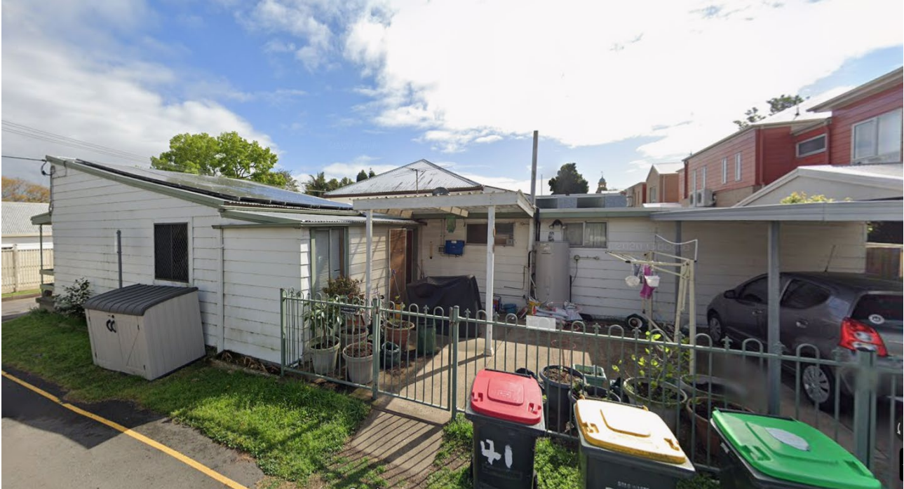
Figure 31: View of the southern-facing façade of 41 Denman Street. There are only three small windows in evidence facing the proposed facility and the dwelling is built on the boundary with no side yard. The outdoor area of the property facing the proposed facility is dominated by a carport, hot water units and pots and plants..
