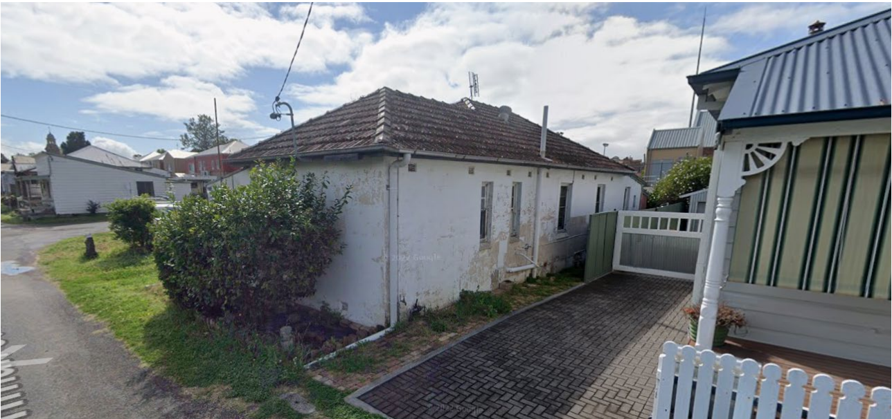
Figure 28: View of the south-facing wall of 46 Denman Street, a property nearby the proposed facility. Several small south-facing windows are in evidence. Given the dwelling is built in close proximity to the property boundary, views are largely dominated by the side of the adjacent dwelling. (Source: Google Maps).
