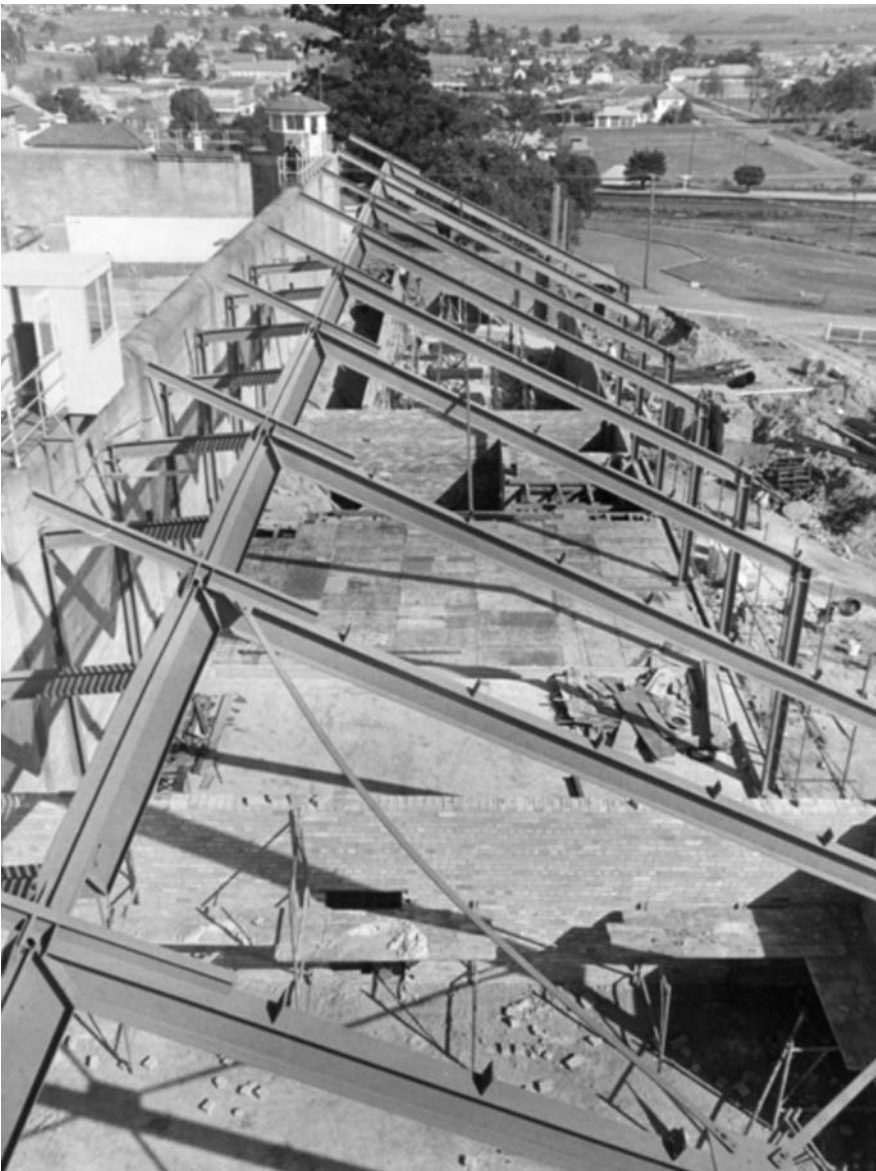
Figure 9 Extensions to Maitland Gaol, reported in Newcastle Morning Herald, July 1975, showing the Store Building (Building 14), subject of the current proposal. source: Hunter Photo Bank, 104 008601.
