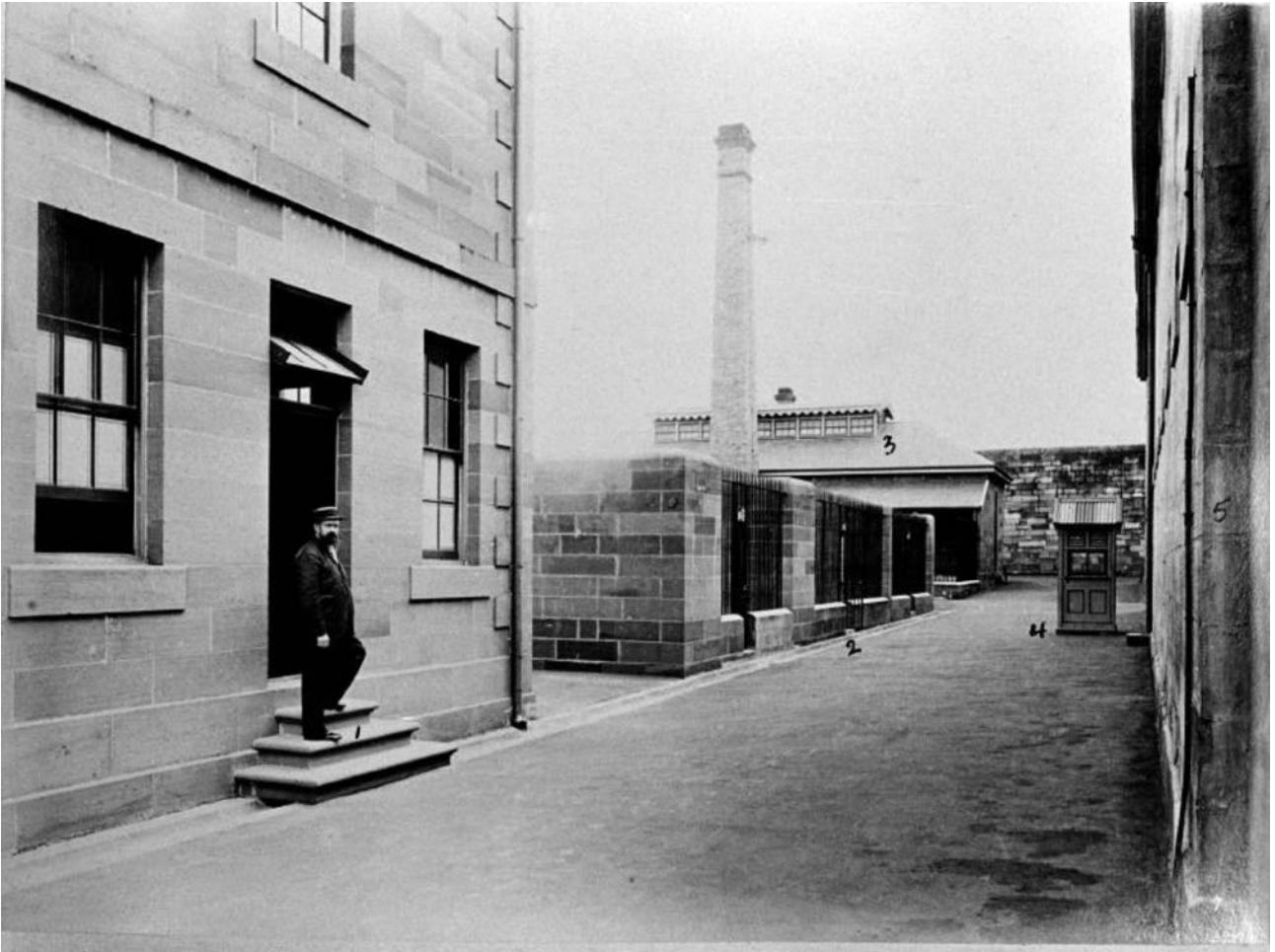
Figure 20 Cookhouse with new chimney stack, gaol office on left, c1897. source: Photographic views of NSW Prisons DOCS.
