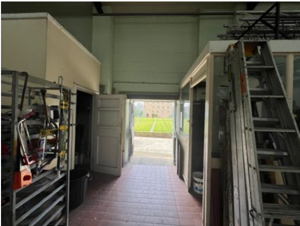
Figure 52 Access to laundry provided via an opening to the original 1839 perimeter wall. source: Heritas, 2022.
