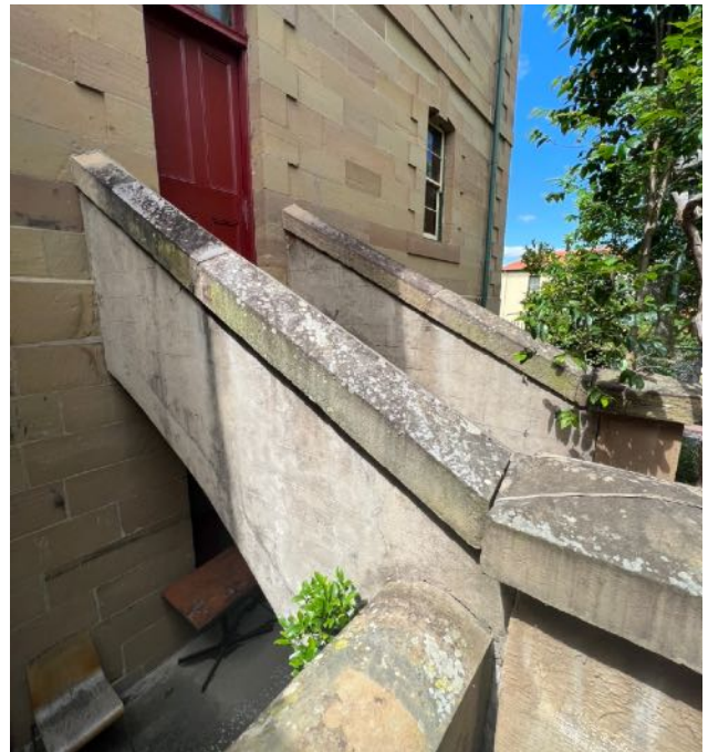
Figure 61 View of patterned wall with sandstone coping to entrance steps. Stone pillars at right. source: Heritas, 2022.
