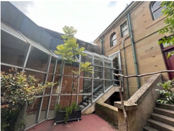
Figure 54 Glazed linkage between the former Amenities Building (now café) and original Lieutenant Governor's Residence. source: Heritas, 2022.
