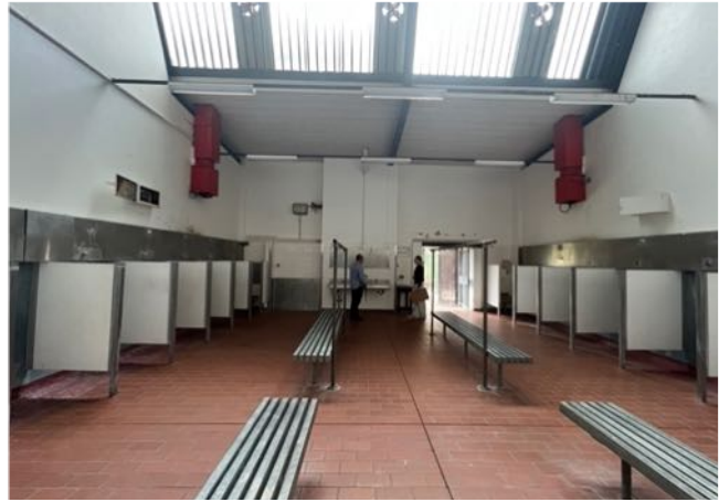
Figure 49 Shower block area with tiled floor finish, rendered wall surface and timber lined raked ceiling. Central seating area with shower partitions lining the internal walls. source: Heritas, 2022.
