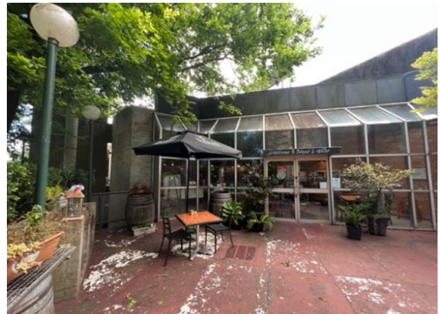
Figure 55 View of former amenities building constructed of brickwork with metal framed glazed entrance portal. Access provided via double doors from the outdoor terrace. Stone perimeter wall to Gaol complex visible beyond. source: Heritas, 2022.
