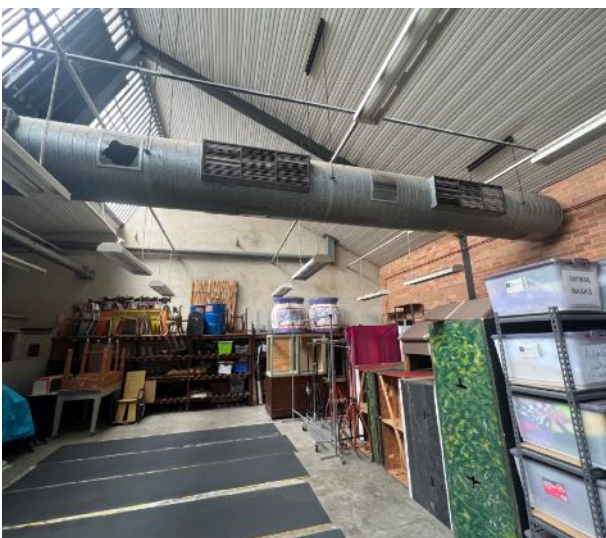
Figure 44 View of Saddlery used as a storage facility. source: Heritas, 2022.
