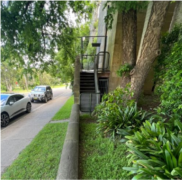
Figure 22 Ravensfield stone retaining wall with curved coping to western boundary. Concrete stairs to 1970s addition beyond. Mass planting bed of Agapanthus and Murraya hedges at right. Café concealed from John Street via the stone wall with dense plantings. source: Heritas, 2022.
