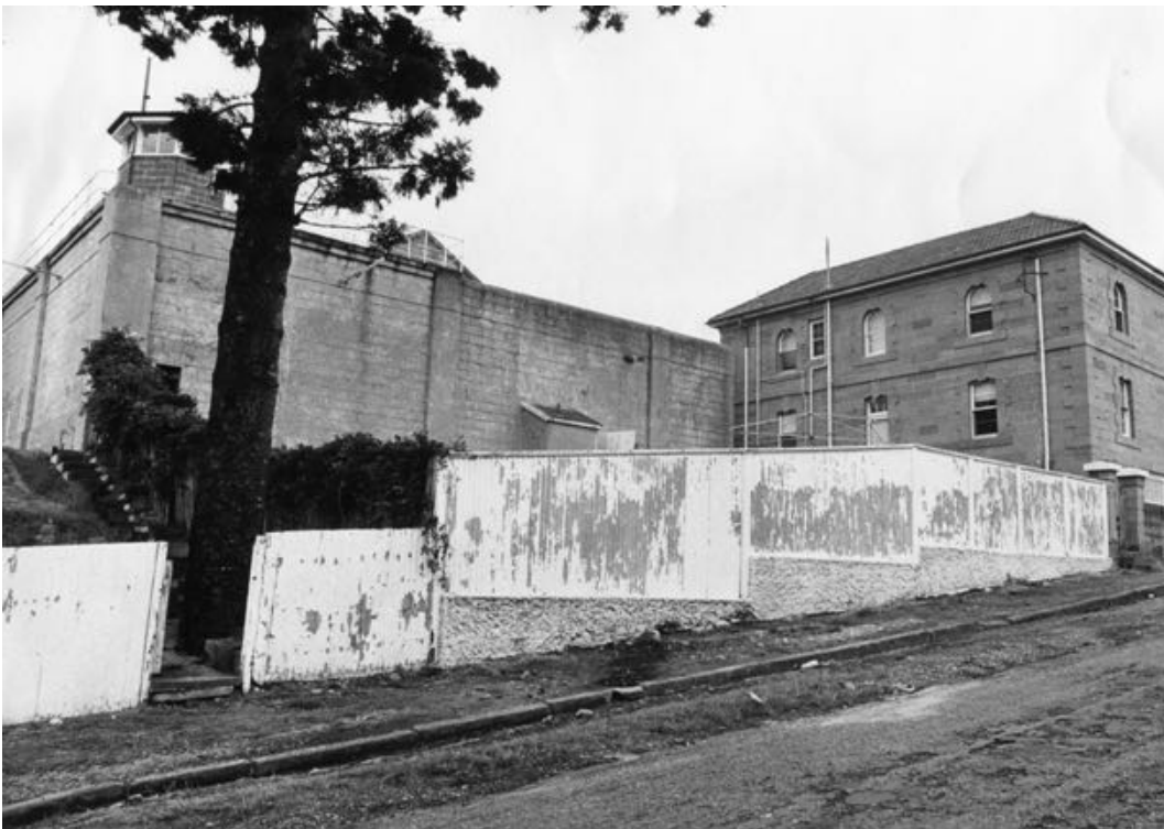
Figure 32 View of Maitland Gaol from the west, January 1974. Depicts gaol wall and entrance prior to construction of the Staff and Warder's Ammenities, now café. source: Hunter Photo Bank, 104 008284.
