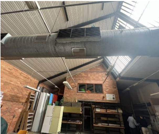
Figure 42 Raked ceiling with clerestory windows and ducting over Saddlery. source: Heritas, 2022.
