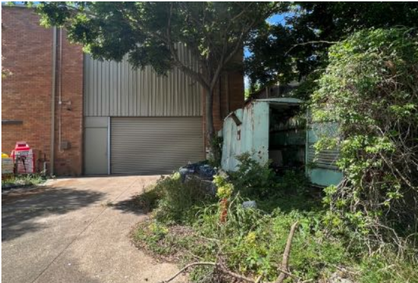
Figure 32 North-west elevation to the brick Store building with metal cladding and metal roller door. source: Heritas, 2022.
