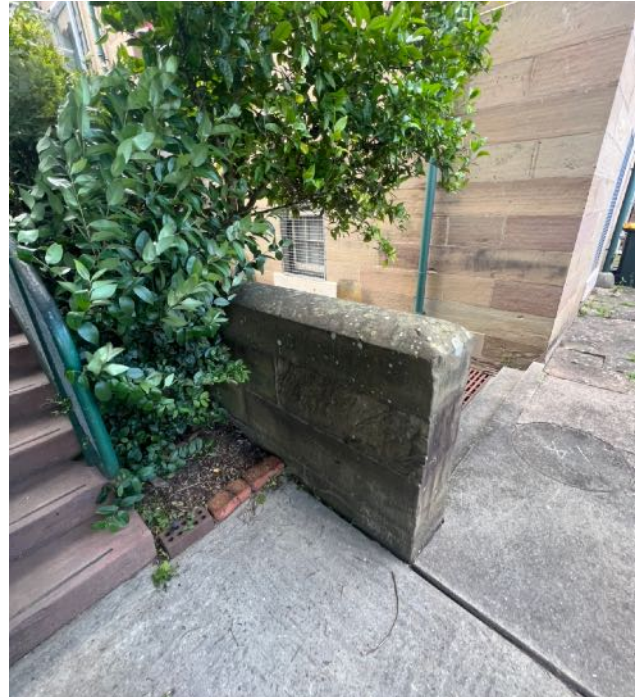
Figure 59 Ravensfield stone wall with curved coping adjacent to the café entrance steps. Ashlar stone façade of the Lieutenant Governor's Residence beyond. source: Heritas, 2022.
