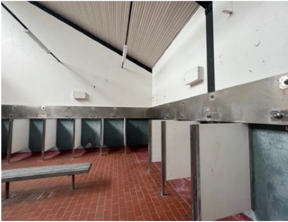
Figure 48 Stall partitions to perimeter of shower block. source: Heritas, 2022.
