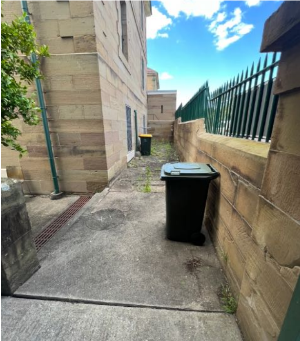
Figure 58 View of ashlar Morpeth sandstone wall to a portion of the John Street boundary with spear topped metal balustrade. Concrete paving to former Lieutenant Governor's Residence surrounds. source: Heritas, 2022.
