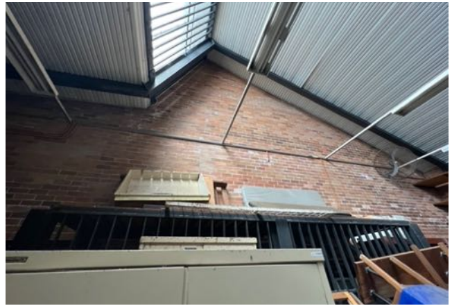
Figure 35 View of exposed brick walls with clear glazed clerestory windows and timber lined raked ceiling. source: Heritas, 2022.
