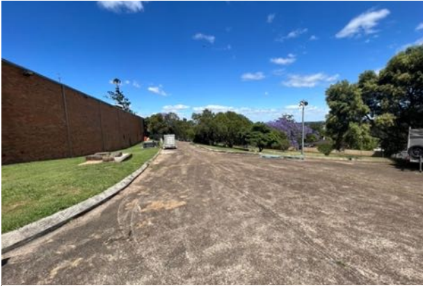
Figure 30 North-west elevation to the 1970s store and workshop building, viewed from the service road. source: Heritas, 2022.
