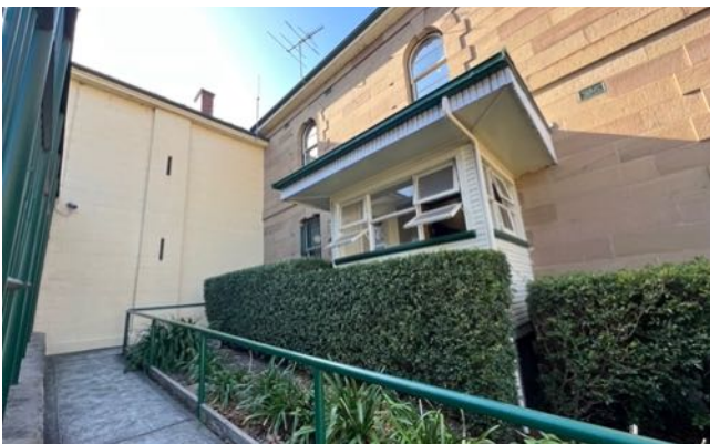
Figure 45 Concrete access ramp with entry alcove at right. source: Heritas, 2023.
