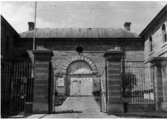
Figure 13 View of Gatehouse with Governor's residence at right, 28 January, 1958. source: Newcastle Morning Herald, Newcastle Library, Hunter Photo Bank, 104 005524.
