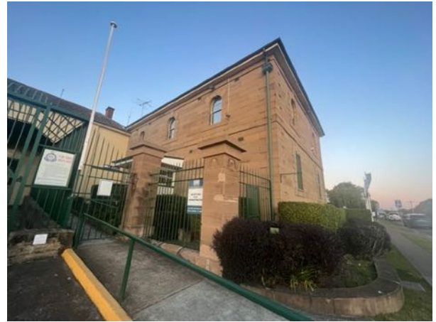
Figure 44 View of sandstone façade with decorative quoins and string course. source: Heritas, 2023.
