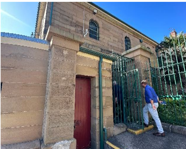
Figure 54 Entry to the Sentry Box, facing north. source: Heritas, 2023.
