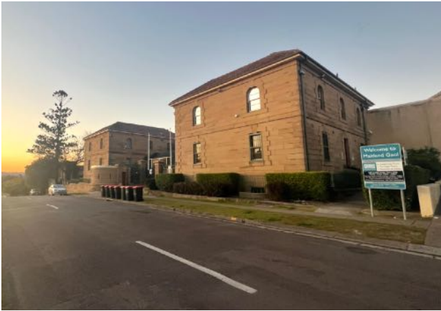
Figure 43 View of former Governor's residence from John Street. source: Heritas, 2023.
