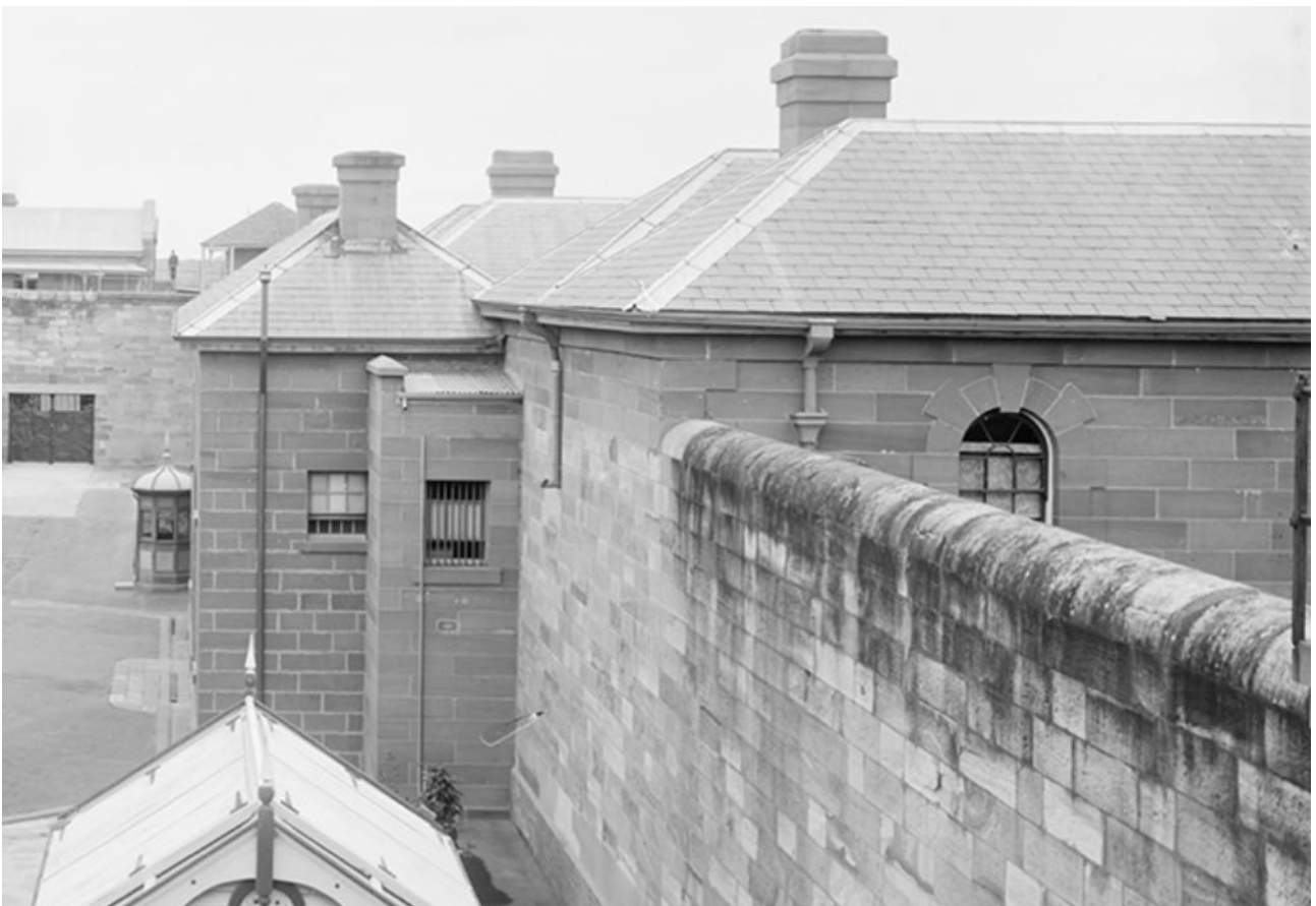
Figure 10 View of former Lieutenant Governor's Quarters and adjoining Gatehouse, undated. source: DPWNSW, SLNSW, NRS-4481-4-206-[AF00198342].
