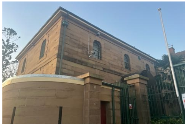
Figure 30 View of quoined arched window openings with sliding sash timber frames. source: Heritas, 2023.
