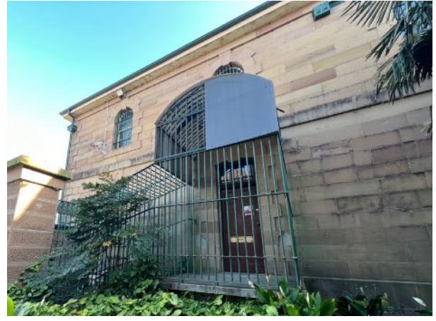
Figure 38 Stone façade with partially clad metal security cage over southern entrance. source: Heritas, 2023.
