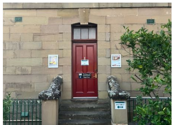
Figure 48 Entrance to southern façade of Governor's residence with quoin doorway and ornamental wall vents. Masonry stairwell with saddleback coping. source: Heritas, 2023.
