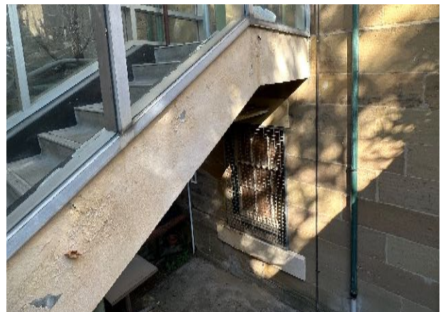
Figure 42 Detailed view of basement window beneath glazed linkage. source: Heritas, 2023.
