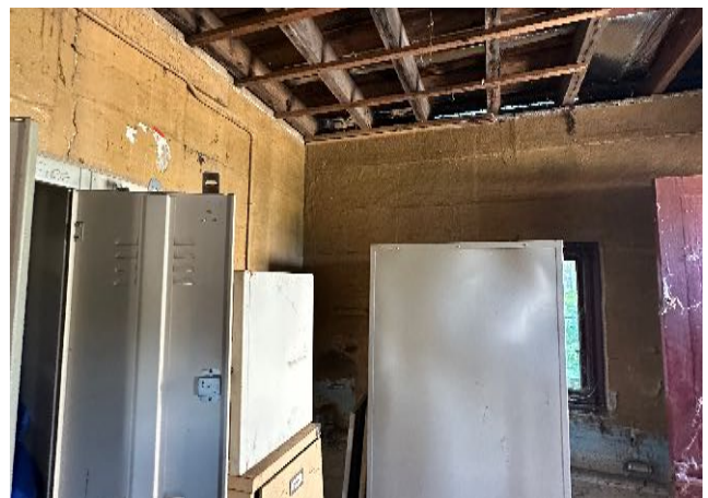
Figure 57 Ceiling removed over Sentry Box. source: Heritas, 2023.
