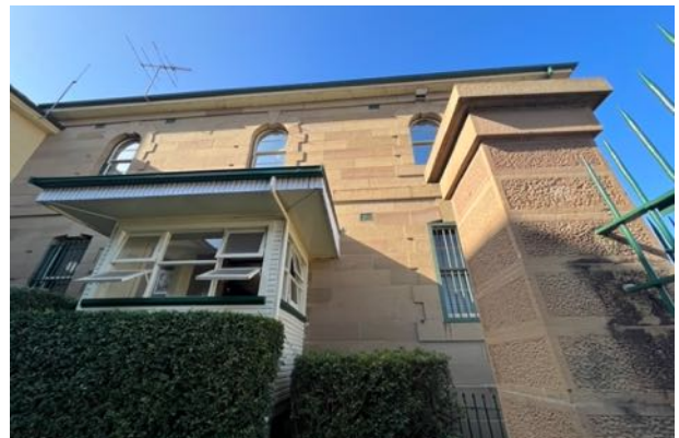
Figure 46 View of northern façade of Governor's quarters with original sparrow-pecked pillar at right. source: Heritas, 2023.
