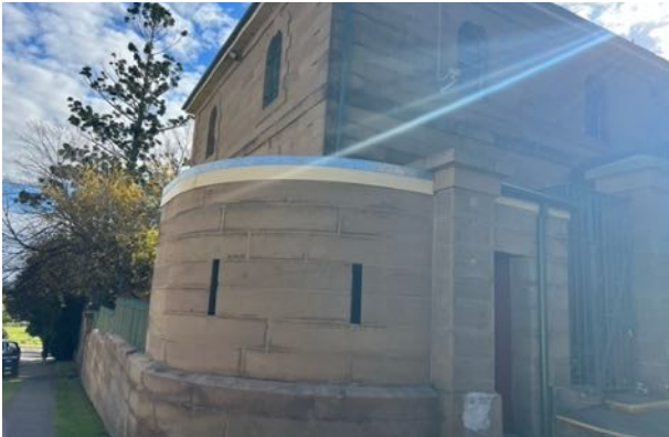
Figure 52 External view of the Sentry Box, facing north, with the Lieutenant Governor's residence behind. source: Heritas, 2023.
