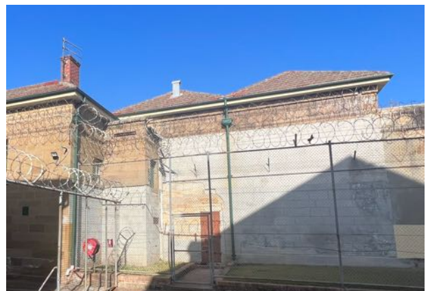
Figure 40 View of access door from ground level of Lieutenant Governor's residence to internal Gaol courtyard. Double hipped tiled roof with original chimneys removed. source: Heritas, 2023.
