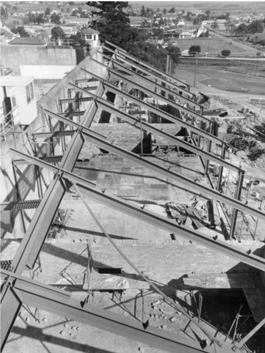
Figure 29 Extensions to Maitland Gaol, by Newcastle Morning Herald, July 1975, showing the Store Building (Building 14), subject of the current proposal. source: Hunter Photo Bank, 104 008601.
