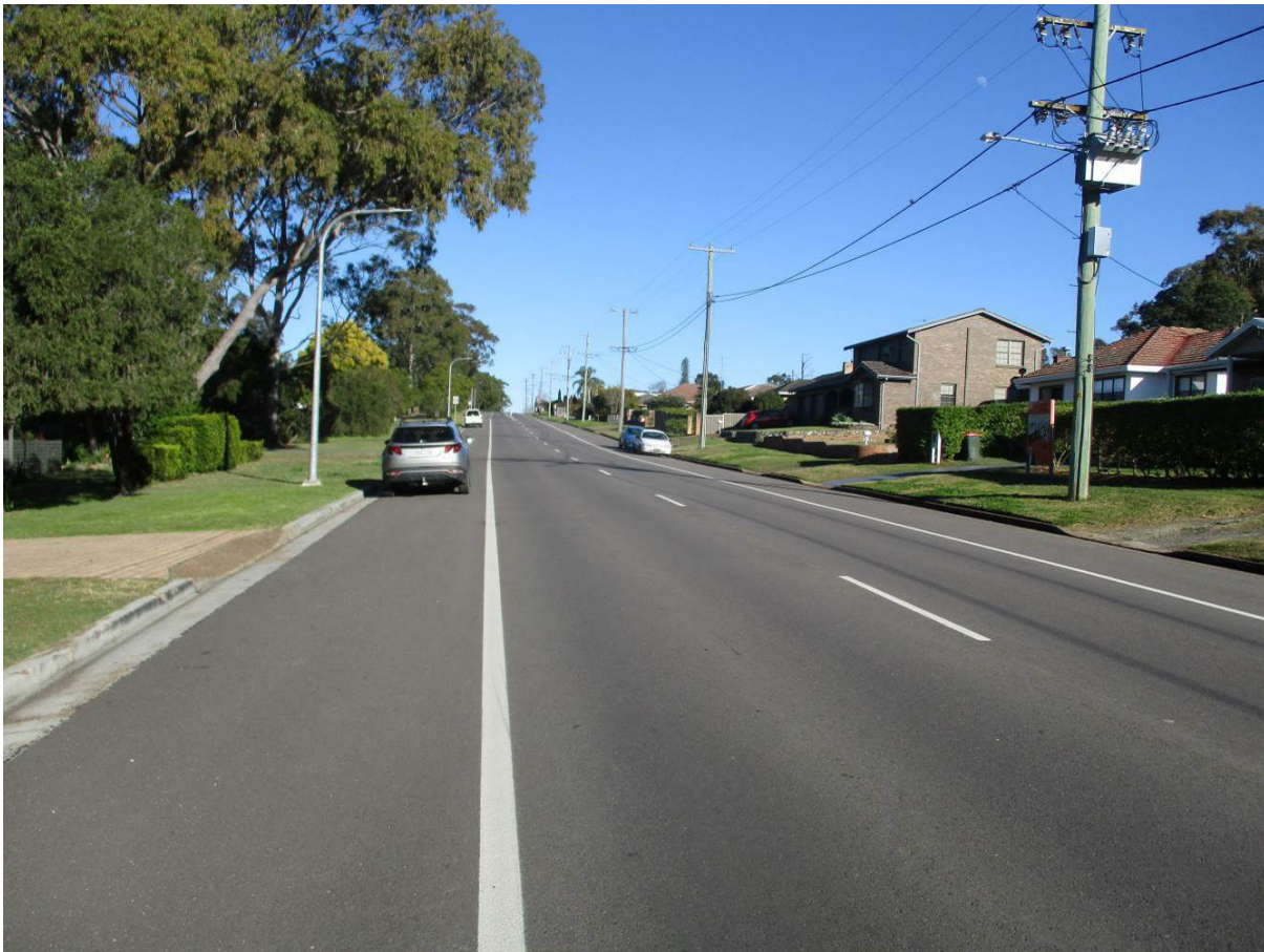
Photograph 2 – Paterson Road along site frontage.
