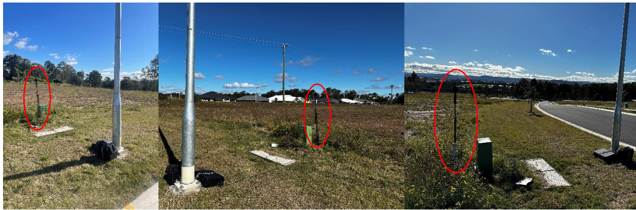
Figure 10 – Logger Installation at 15 Loane Circuit, Farley
