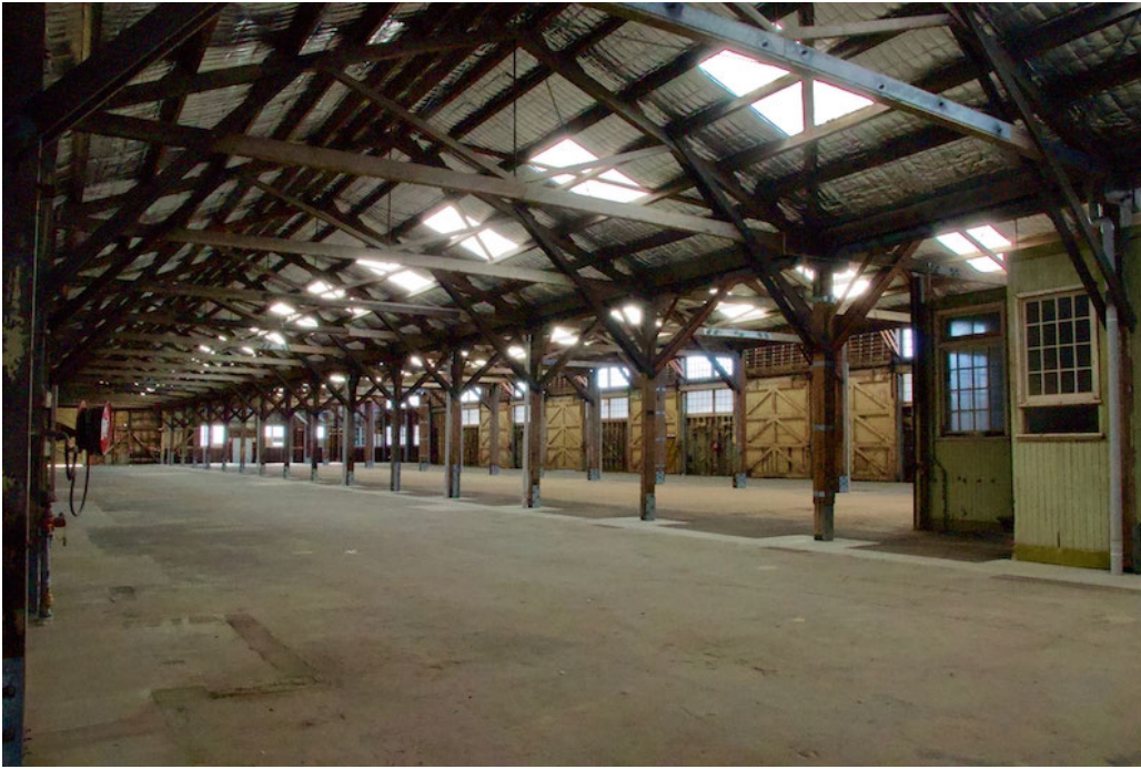
Wooden poles and beams
