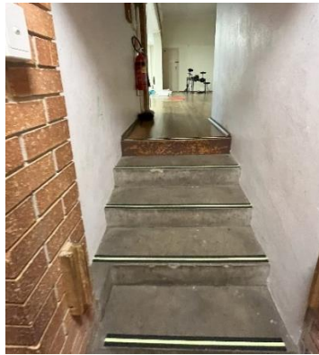
Figure 7: Existing Stage Stairs
