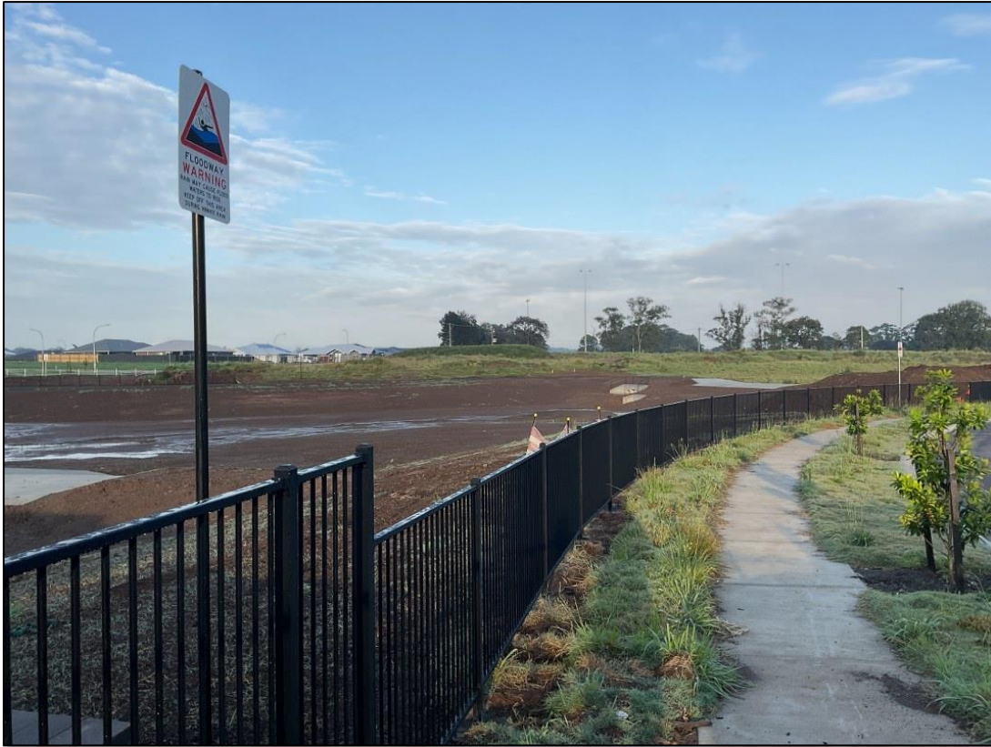
Plate 5 (P5) Water retention basin and partially manage grasslands to the south-west
