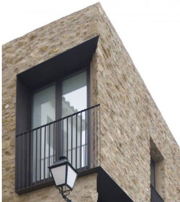
Figure 3-116 Contrast texture with sharply defined openings and fine steel balustrades
