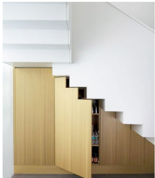
Figure 3-85 Storage space under stairs
