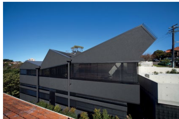
Figure 3-106 Interesting roof forms and integration of privacy and sun control devices to overall building design
