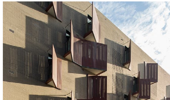
Figure 3-92 Angled privacy screens direct views away from the side boundary. They could also include bay windows
