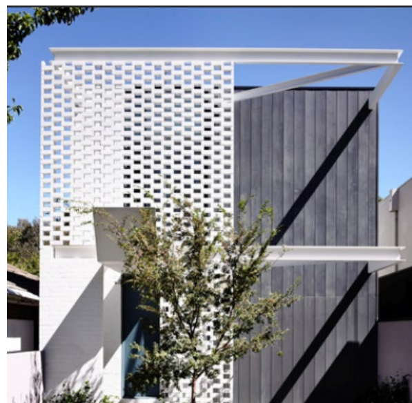
Figure 3-93 Privacy screens are integrated into the facade and provide part of the architectural expression
