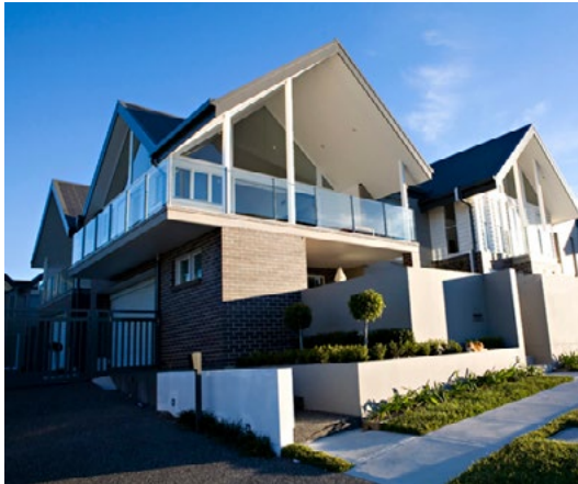
Figure 3-108 Roof form expressed
