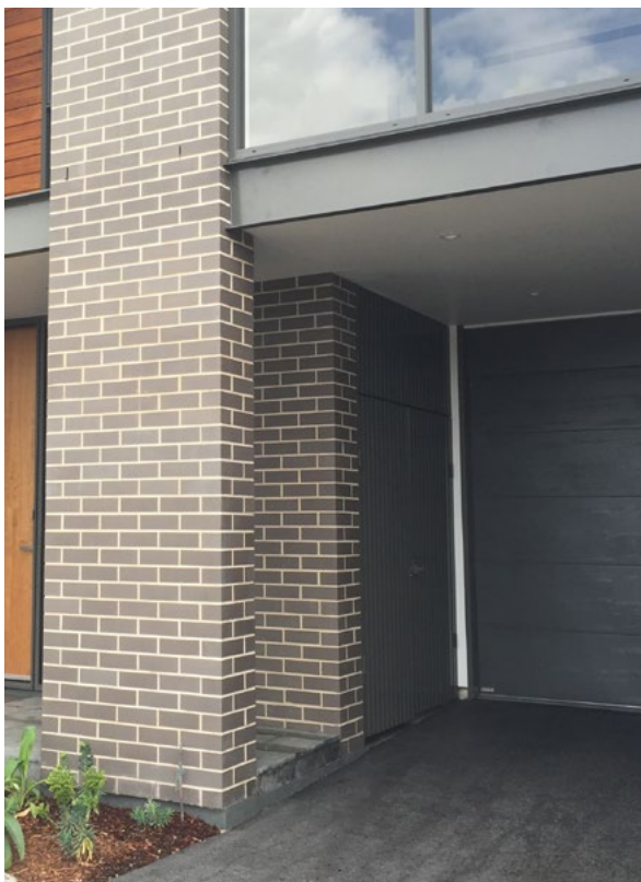
Figure 3-134 Provide bin areas that are screened and incorporated into the landscape or building design
