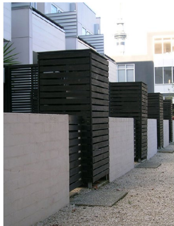
Figure 3-135 Bin areas fronting the street can be designed and incorporated into the building or landscape elements
