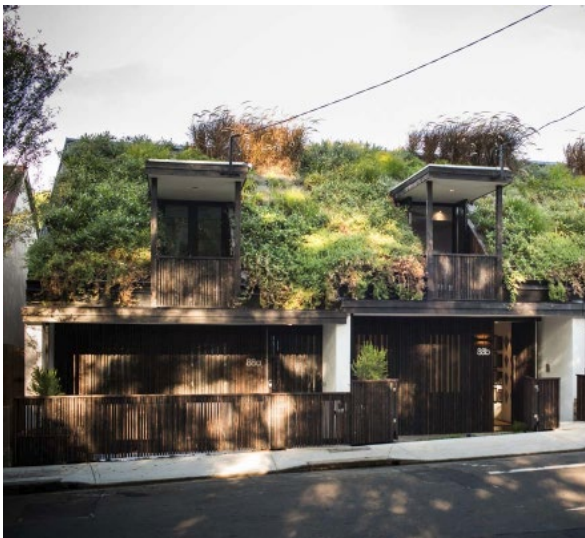
Figure 3-39 Green roof on terraces
