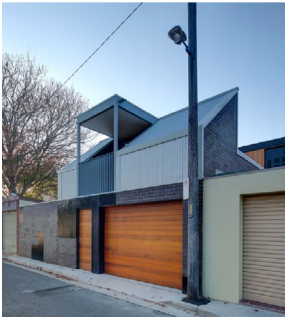
Figure 3-123 Rear outbuildings such as studios should be orientated to the lane to allow for passive surveillance and security
