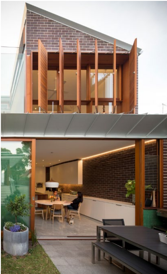
Figure 3-127 Adjustable screens allow control of sunlight
