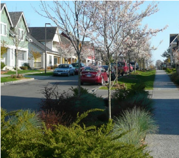
Figure 3-129 Swales can be attractive, and are able to filter and collect the stormwater
