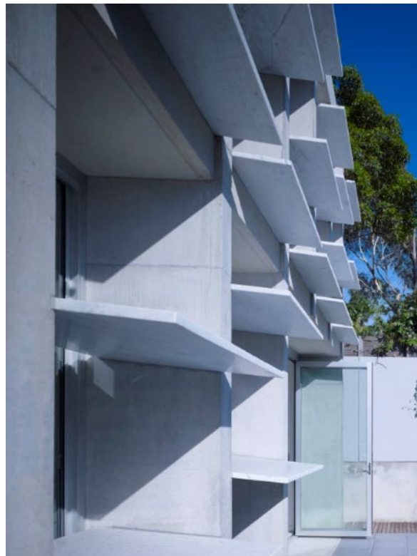
Figure 3-125 Light shelves can reflect sunlight deeper into rooms and provide shade from summer sun
