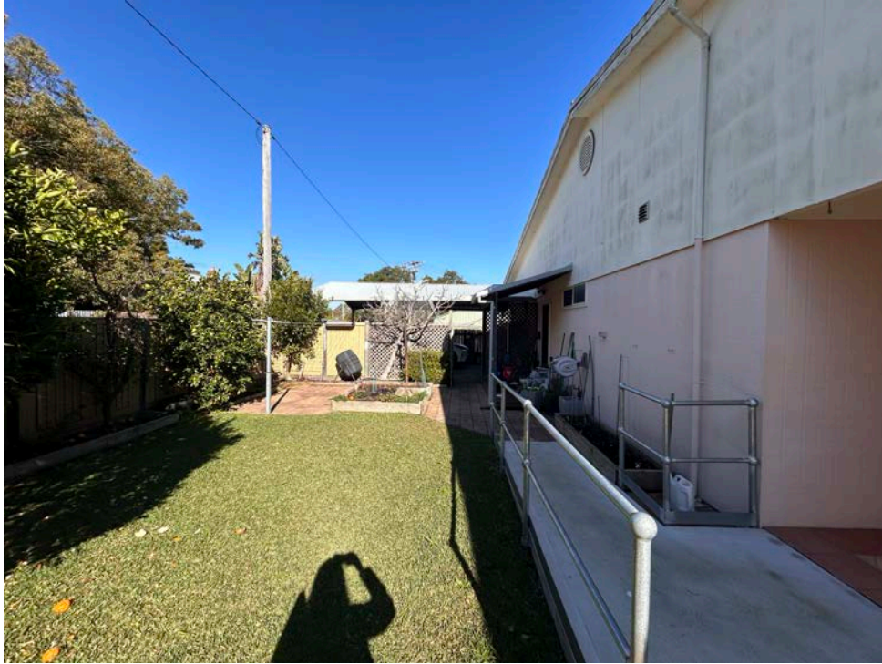
Figure 5: Existing Rear of 73 Bulwer Street (Source: Hoover Group)
