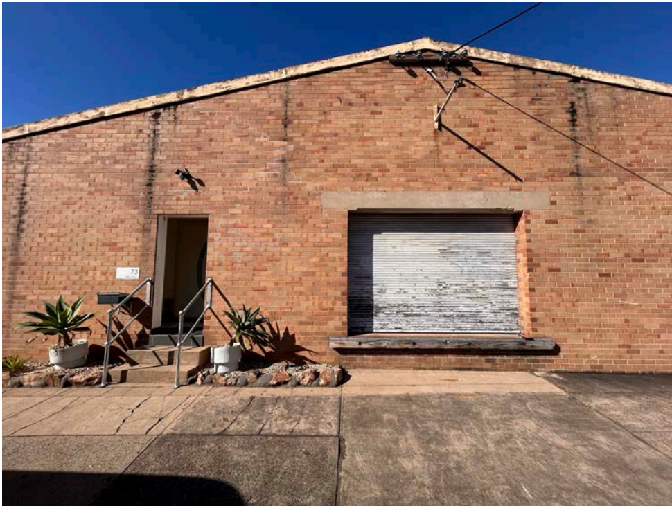
Figure 3: Existing Front Facade of 73 Bulwer Street (Source Hoover Group)
