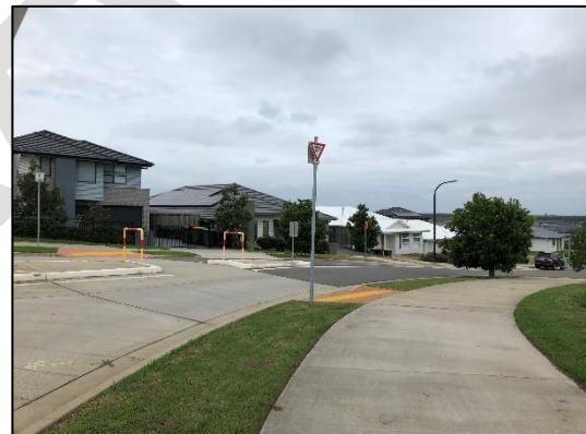
Image 8: Pedestrian infrastructure, including pathway, pedestrian crossing opportunity and refuge island.
