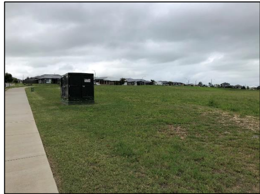
Image 12: View of existing electricity servicing box on project area, located to the west
