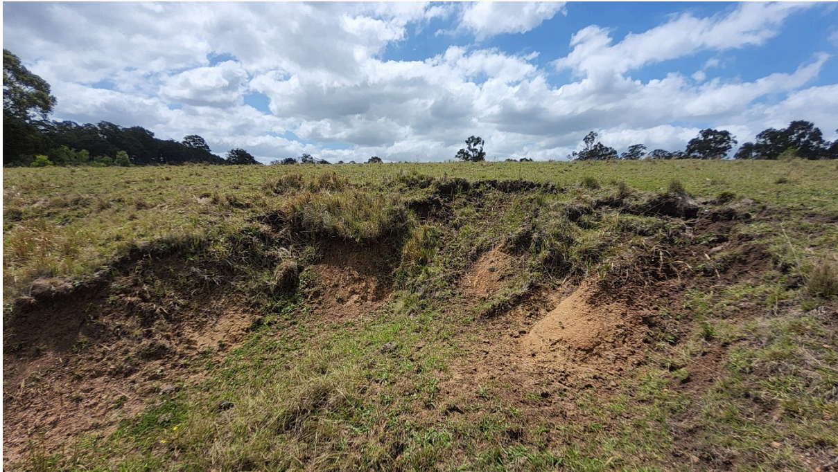
Plate 5. Eroded area adjacent to dam, view to north-west. (Source: Heritage Now 2024)
