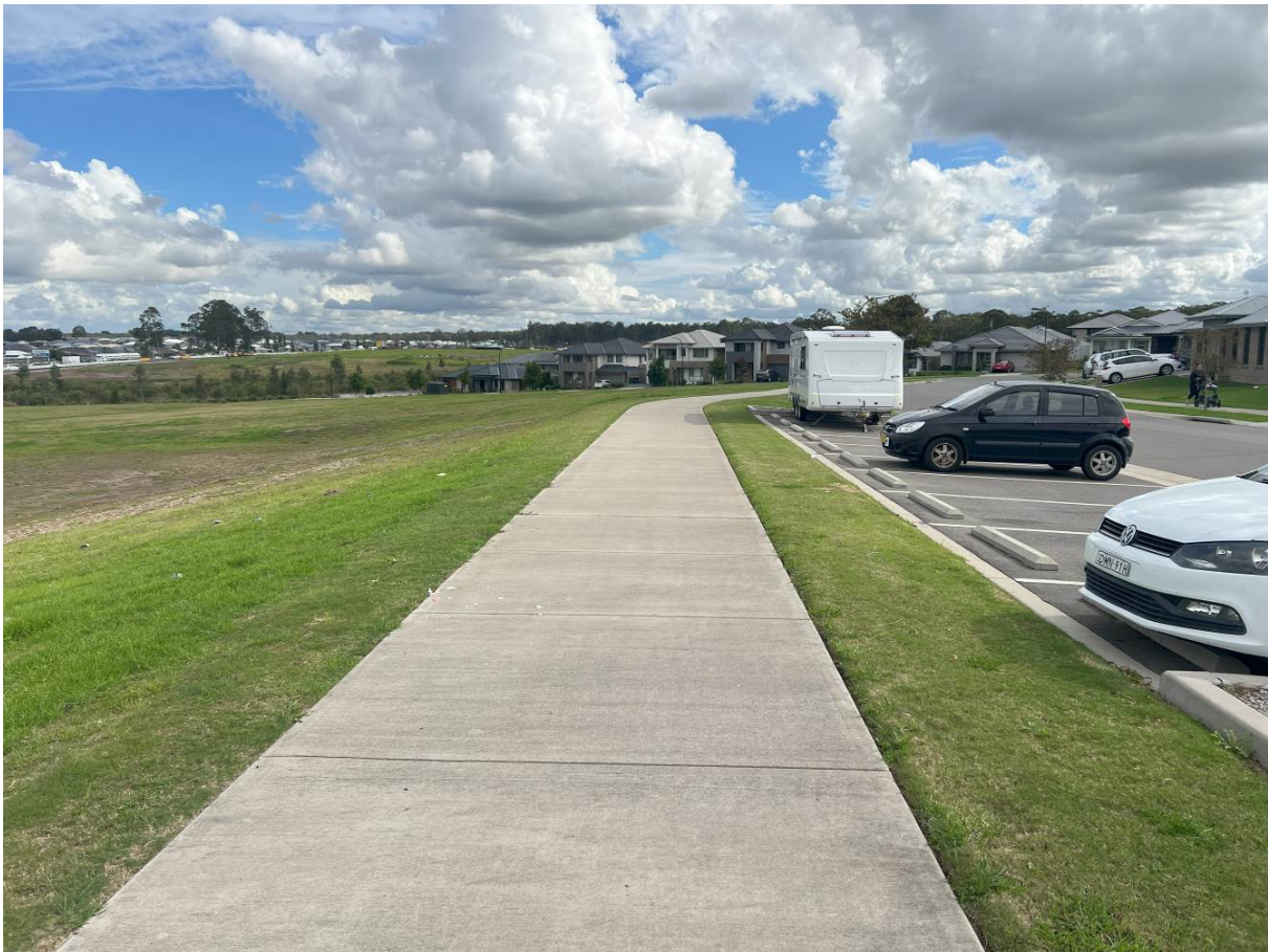
Photograph 7 – Shared Pedestrian / Cycle pathway Suncroft Street.
