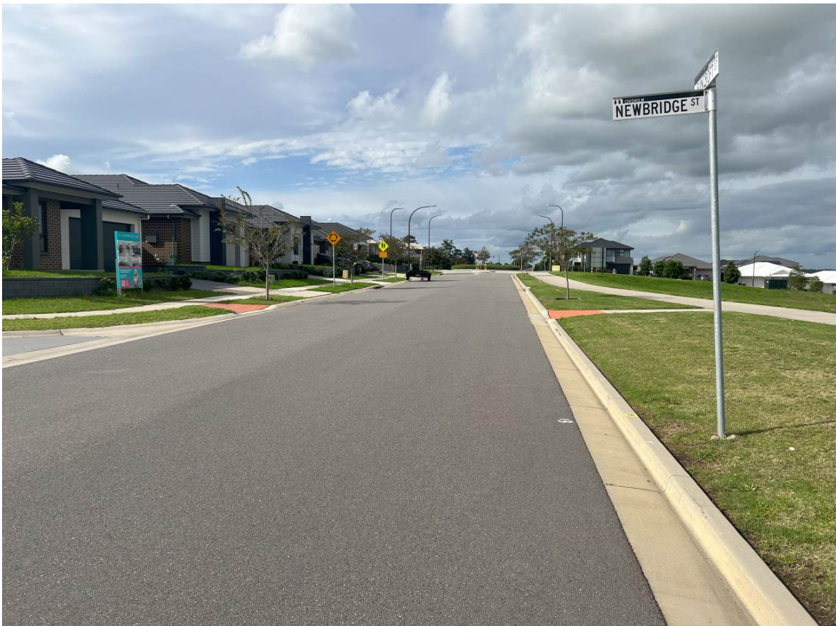
Photograph 6 – Suncroft Street along site frontage.
