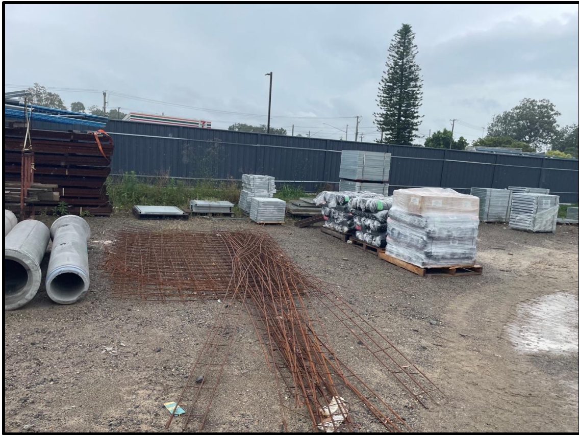
Figure 28 & 29. Concrete piping and pits, as well as other construction materials stored onsite.
