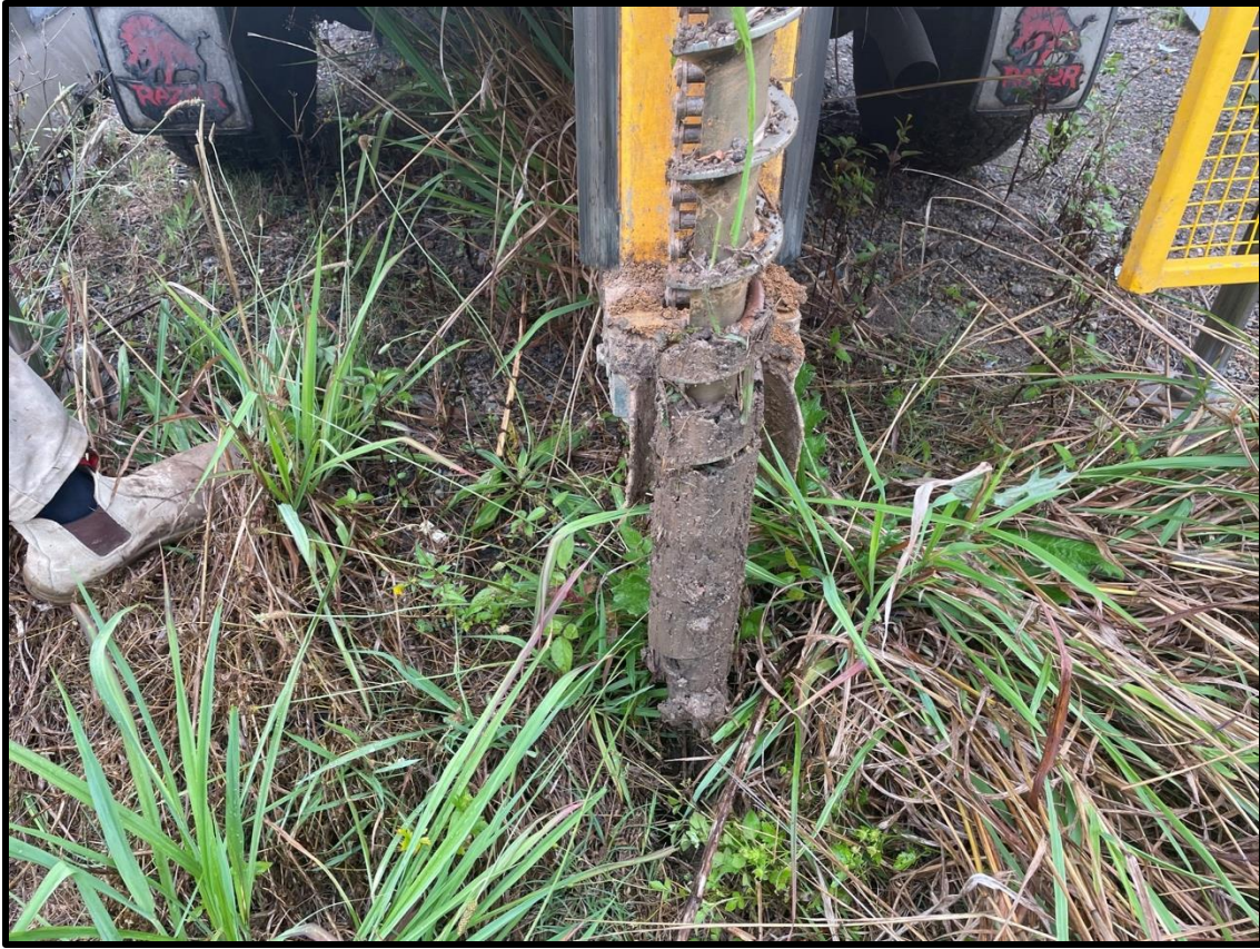
Figure 24. Fill layer encountered in BH2.
