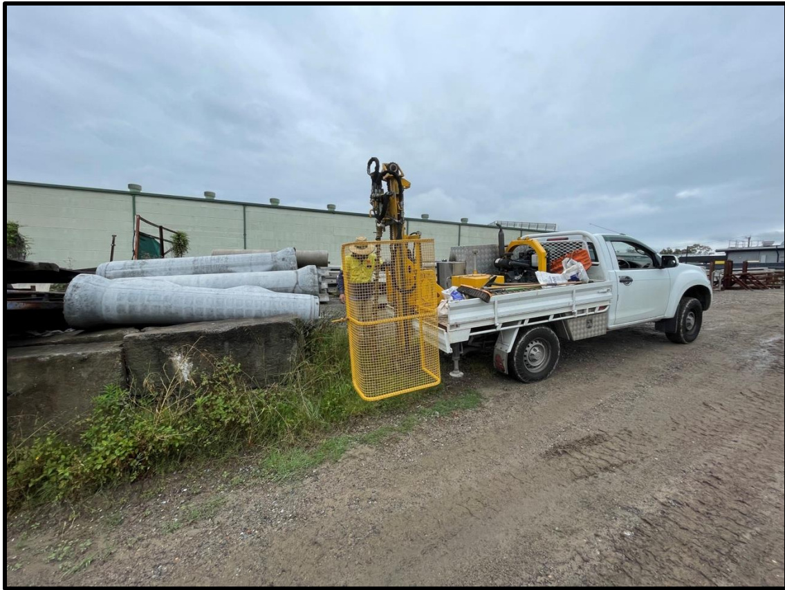
Figure 26. Drilling of BH3.
