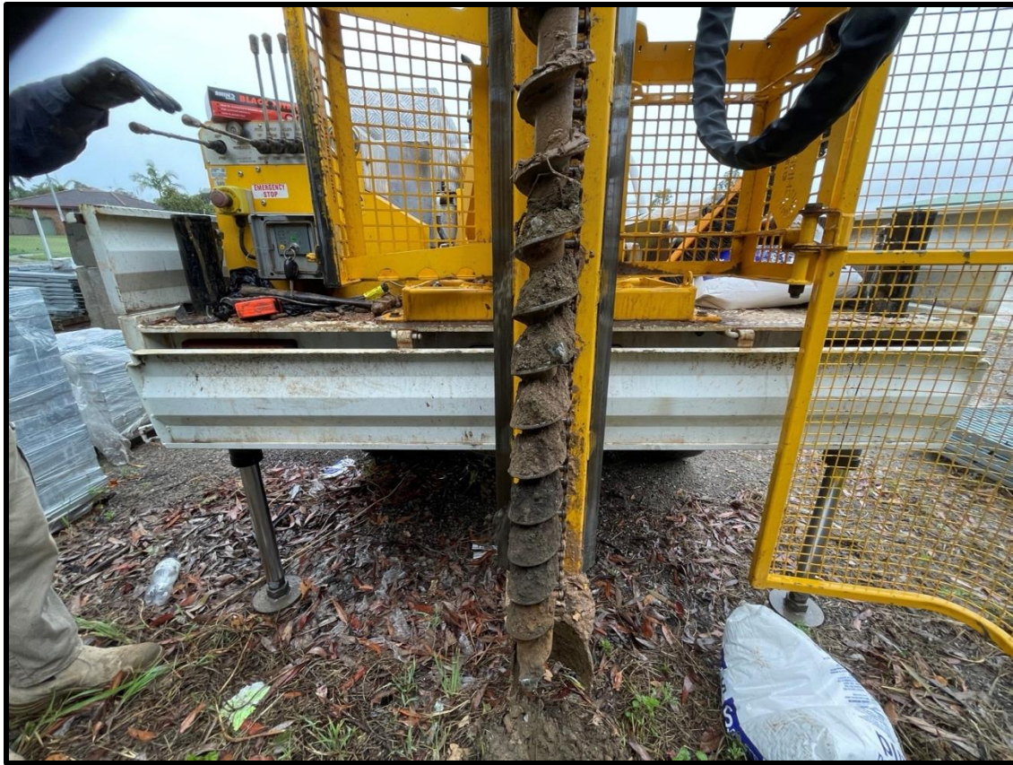
Figure 22. Fill material identified in BH1.
