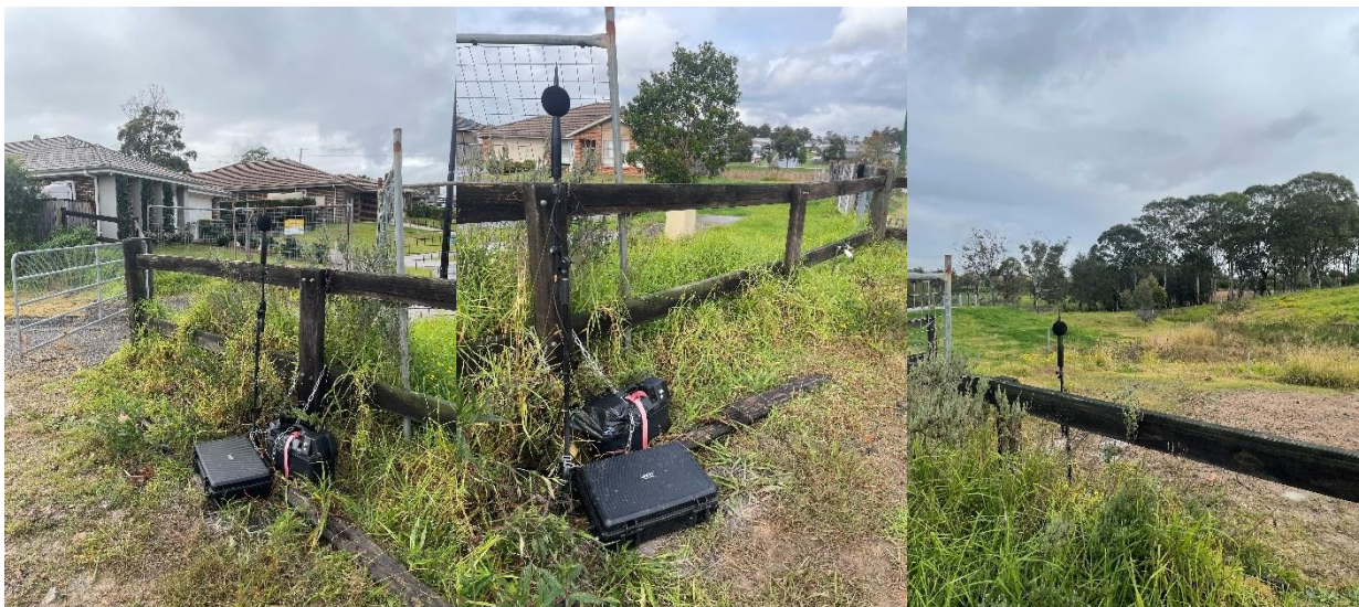
Figure 7 – Logger Installation at 14 Lavender Close, Gillieston Heights
