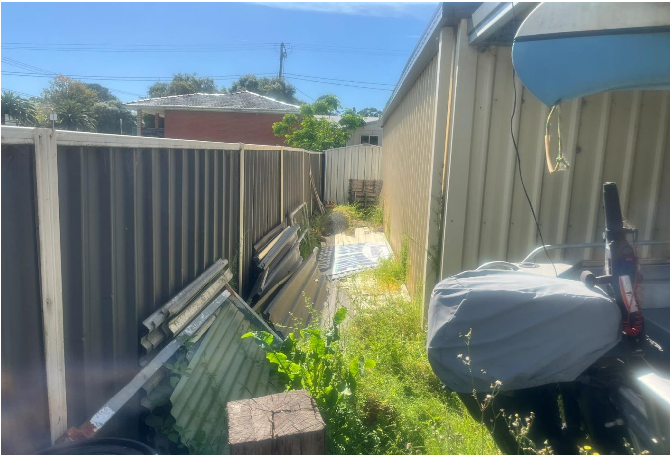
Photograph 24 - Showing northern side of Shed 2.
