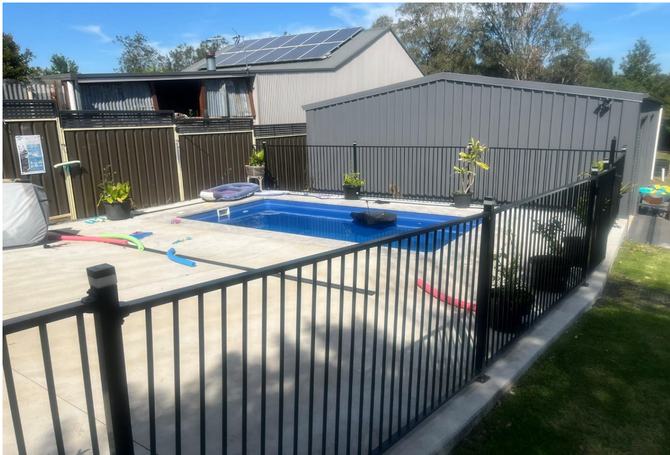
Photograph 34 - Showing swimming pool and concreted area on Lot 3.
