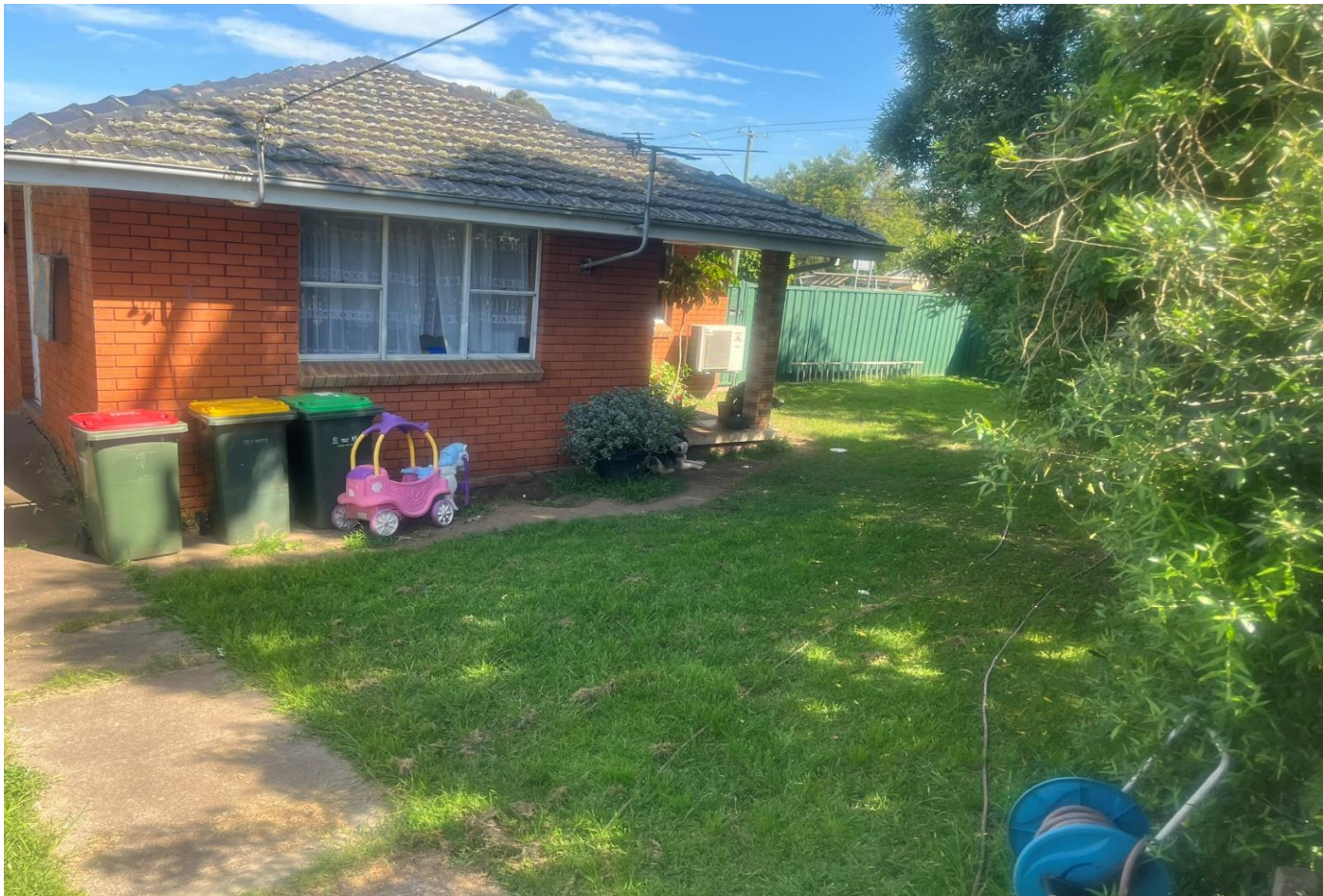
Photograph 2 - Showing the eastern side of Dwelling 1.
