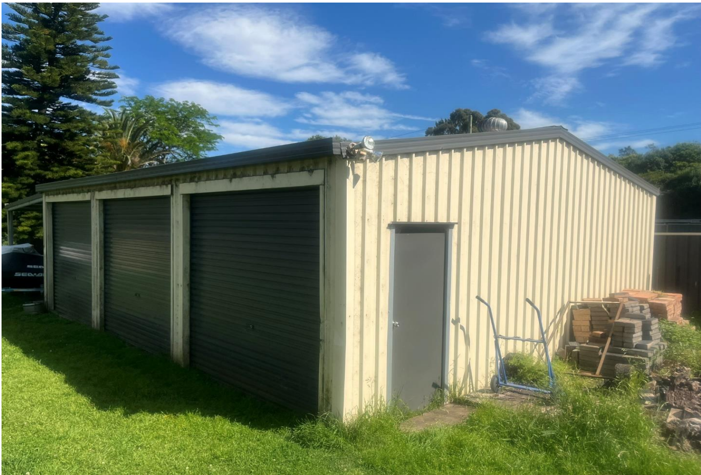
Photograph 22 - Showing Shed 2 on Lot 2.
