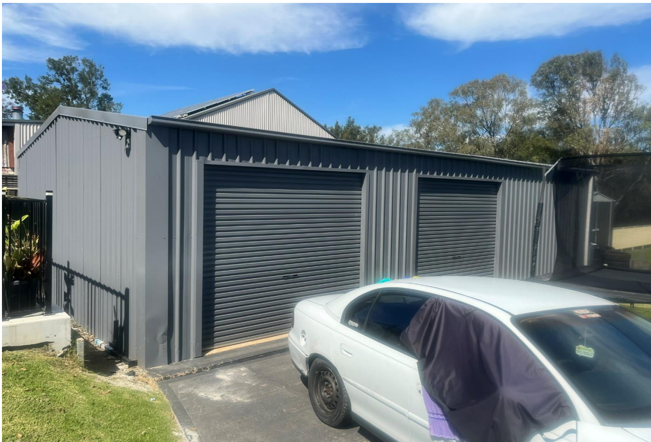
Photograph 35 - Showing Shed 6, vehicle and trampoline on Lot 3
