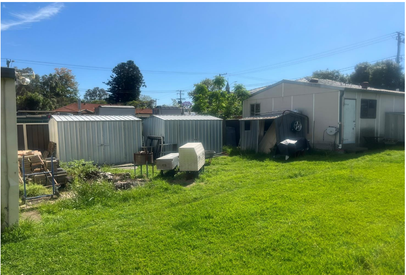
Photograph 21 - Showing Sheds 3, 4 and 5 on Lot 2.
