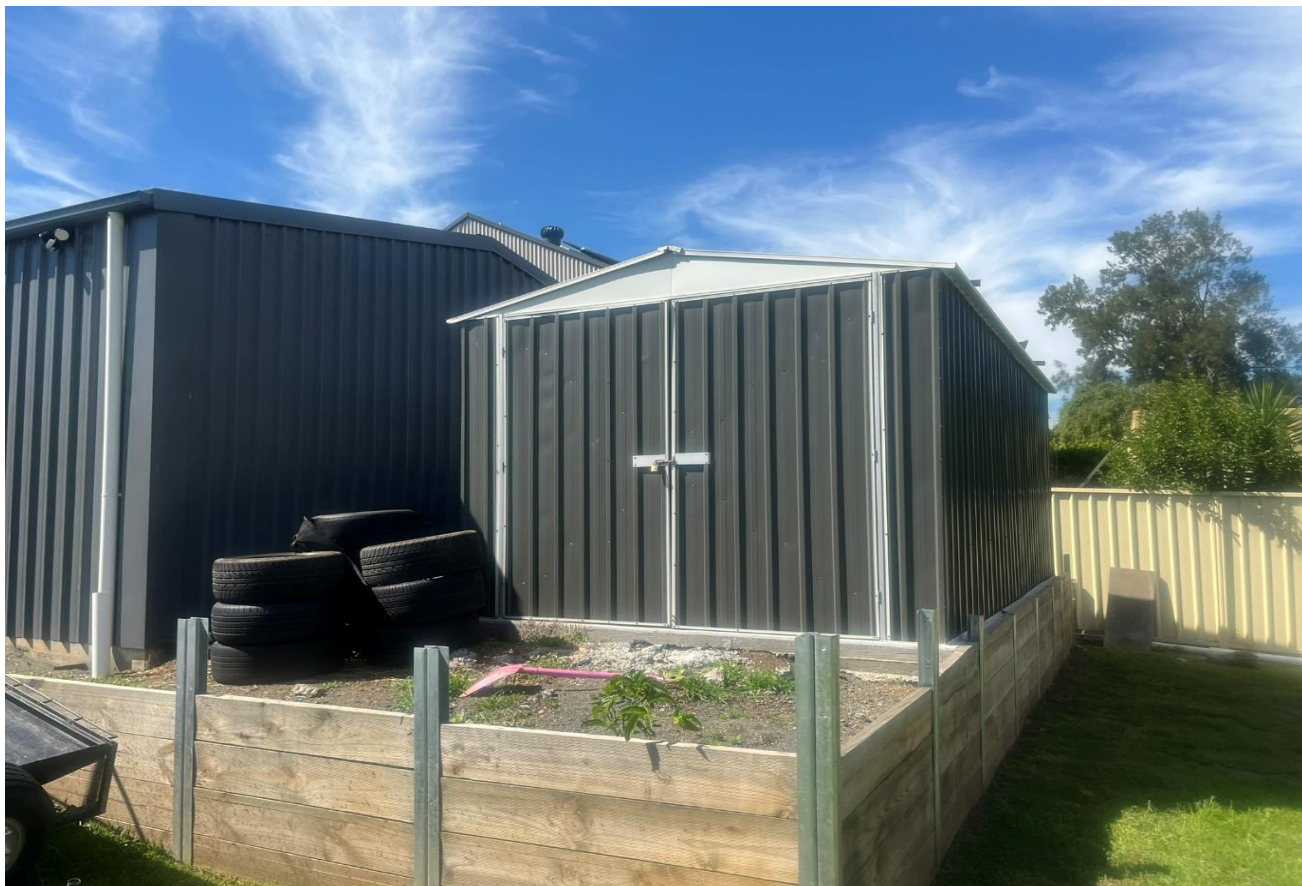
Photograph 36 - Showing Shed 7 on Lot 3
