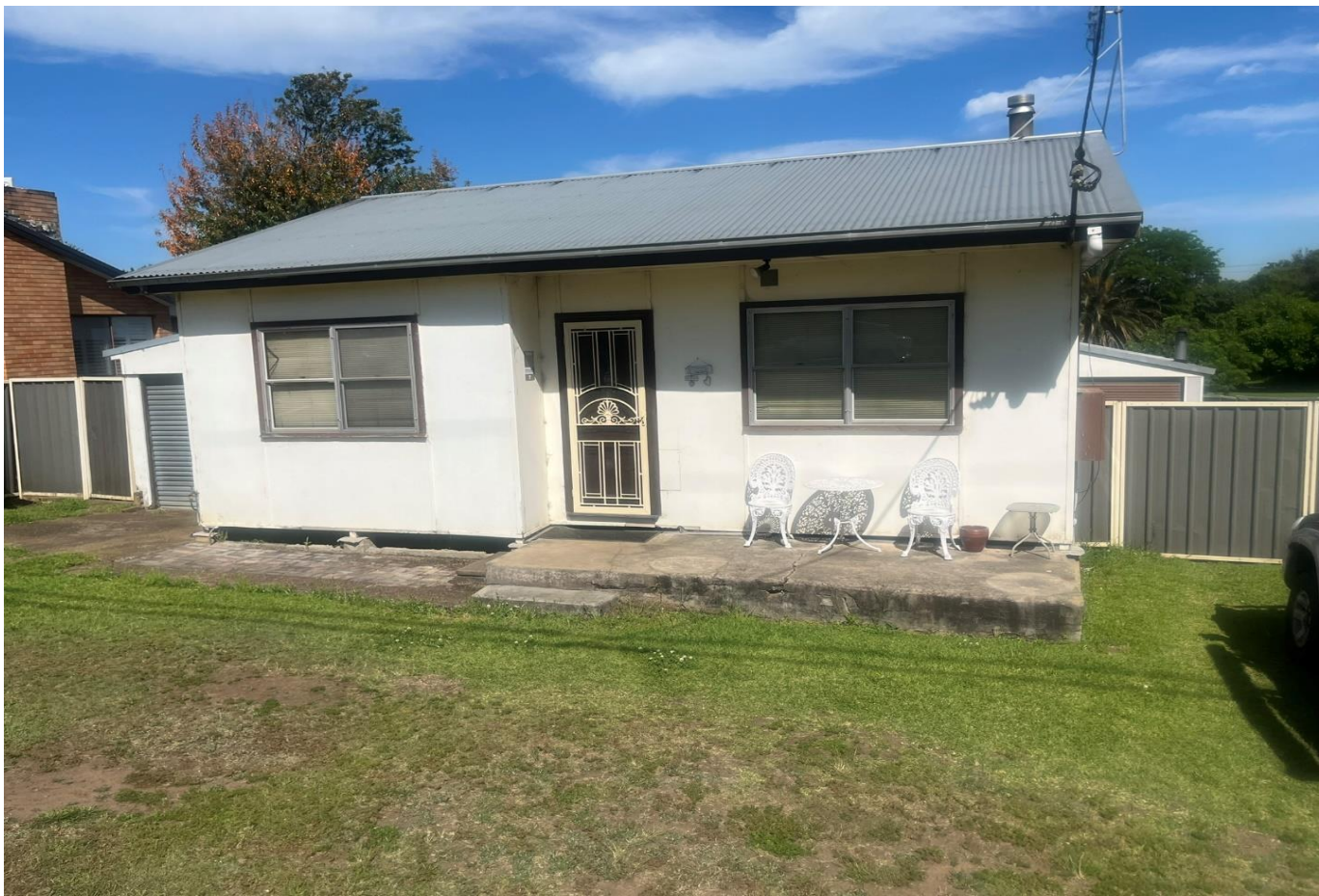
Photograph 13 - Showing the eastern side of Dwelling 2.
