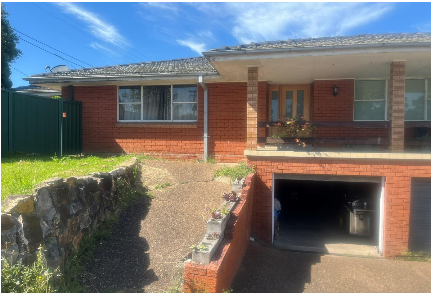
Photograph 1 - Showing northern side of Dwelling 1.
