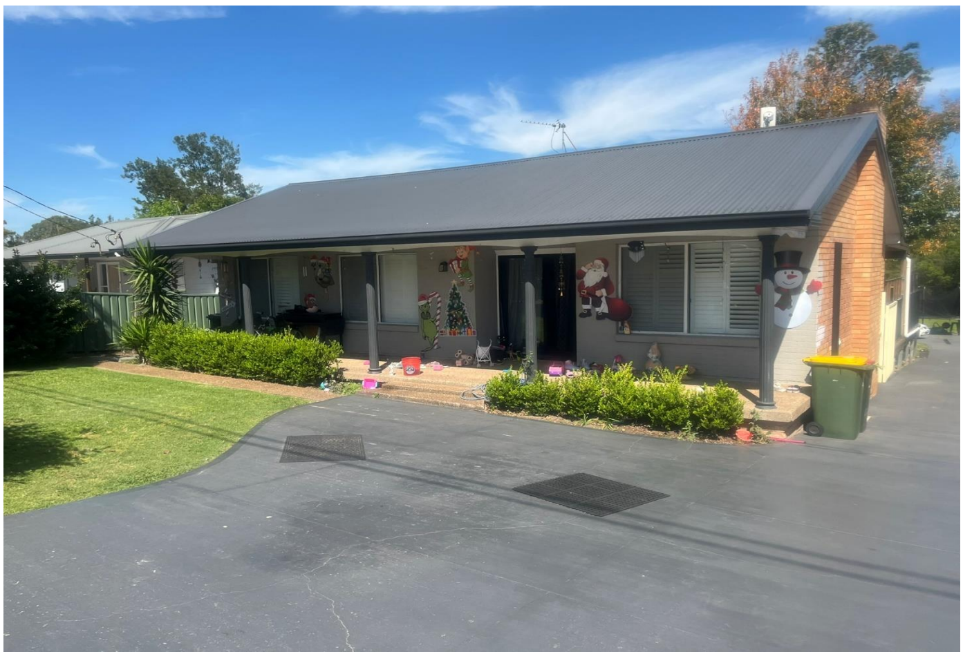
Photograph 31 - Showing eastern and northern side of Dwelling 3.
