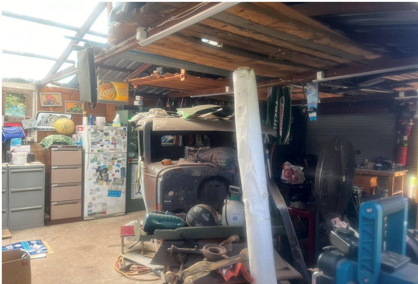
Photograph 20 - Showing interior of Shed 1.
