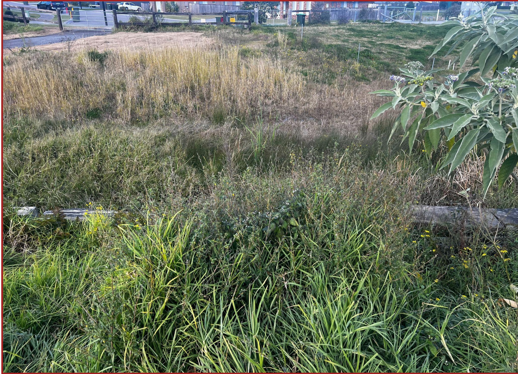
FIGURE 16 Concrete edging on the side of easement running through the middle of the site.
