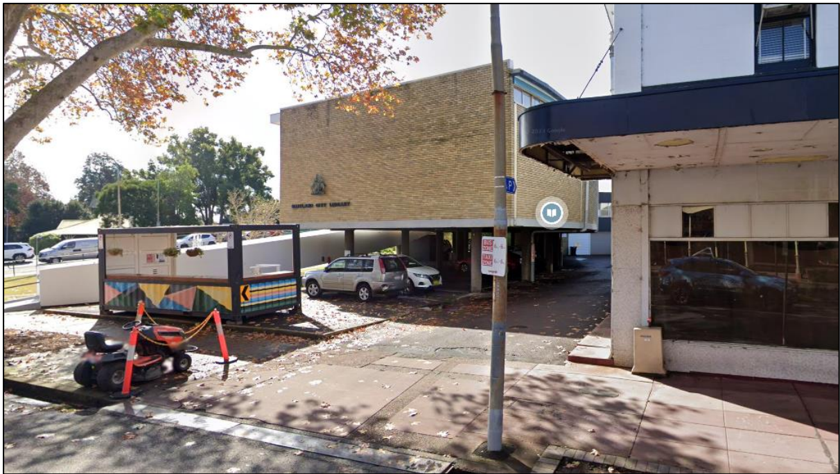
Figure 6: No. 480 High Street, Maitland as viewed from the street (Google Maps 2024).
