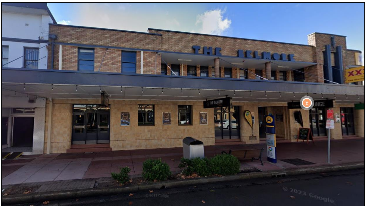
Figure 7: No. 476 High Street, Maitland as viewed from the street (Google Maps 2024).
