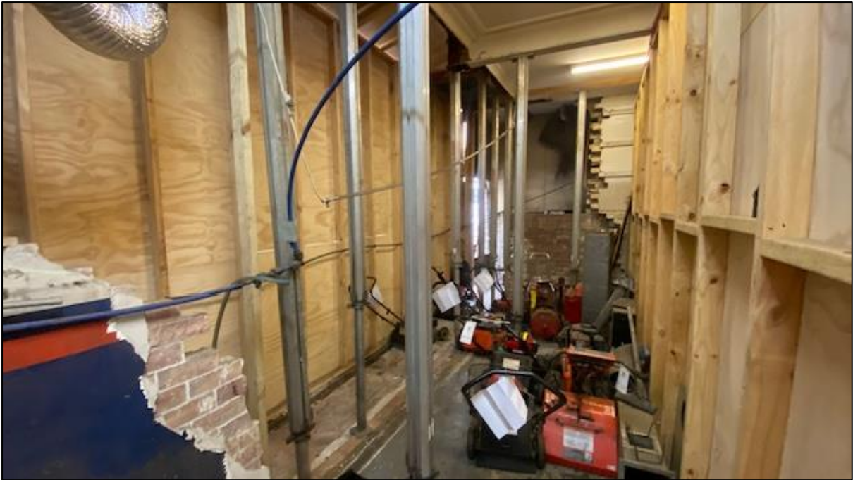
Figure 4: External staircase as viewed from the side of the building adjacent to the northern boundary (Corona Projects 2024).
