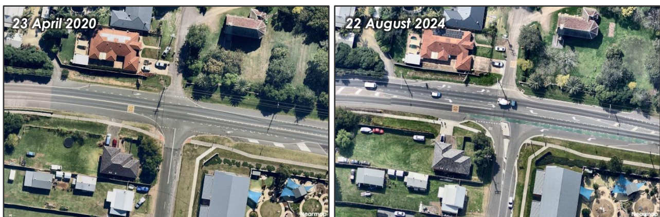
Figure 7 New England Highway / Station Lane Intersection Upgrade
