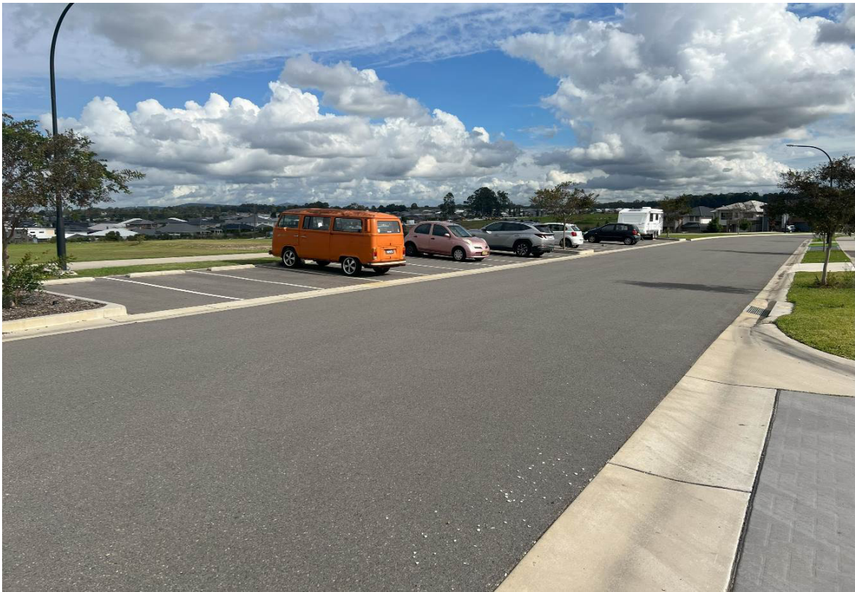
Photograph 3 – Existing 20 space indented on-street car parking bay Suncroft Street.
