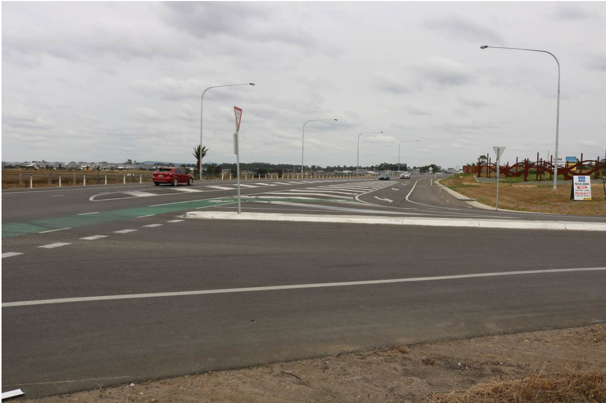
Photograph 4 – Raymond Terrace Road near site.
