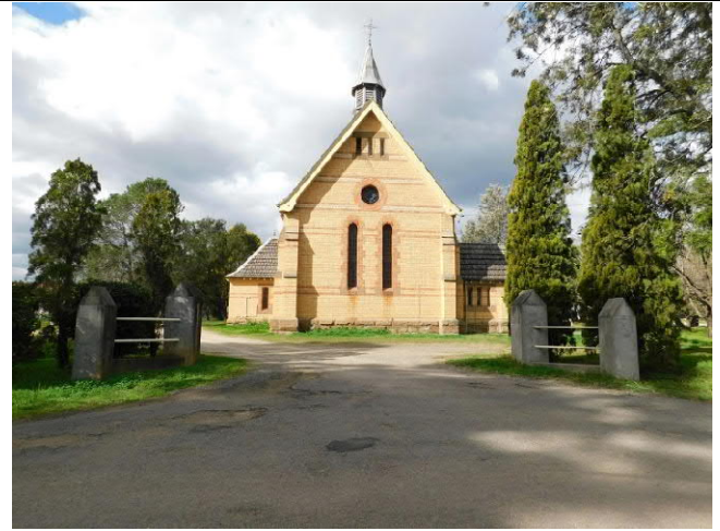
Figure 28: The west façade of the Holy Trinity Anglican Church looking east from Cantwell Road between the gateposts which were installed c1988.
