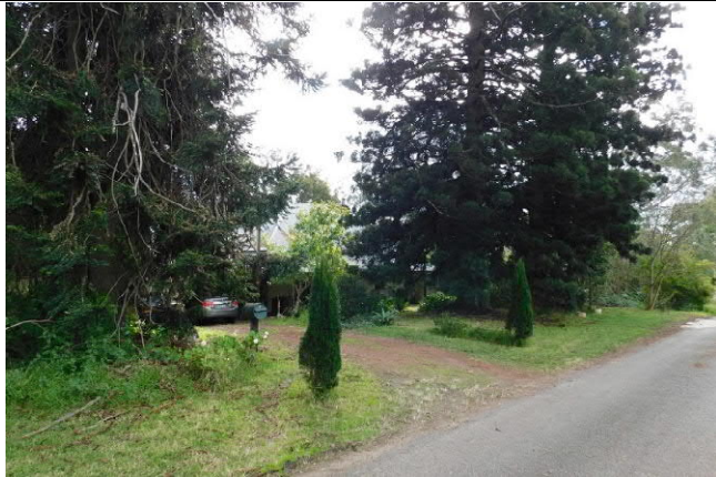
Figure 31: Looking toward Victoria House (Nowland's Lochinvar Coach House) from Cantwell Rd. The building is set back from the road but the landscaping extends right up to it.
