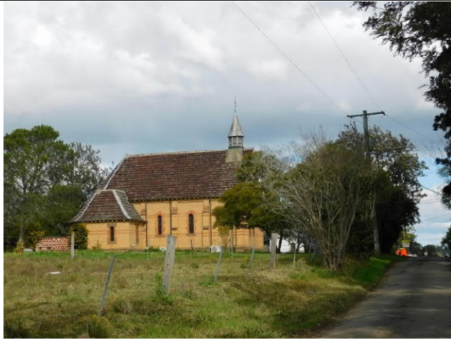
Figure 27: The north side of the Holy Trinity Anglican Church looking south from Cantwell Road. The intersection of the New England Highway is just beyond the trees.
