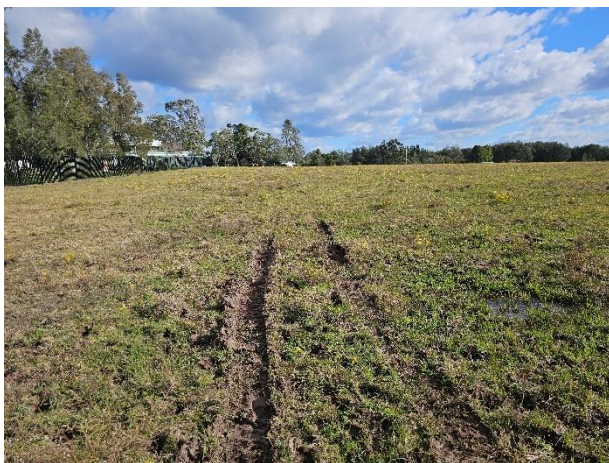
Photograph 7: Facing southwest from near TPQ12. Showing Excavator tracks formed within area of soft / moisture affected ground surface, localised ponded water.
