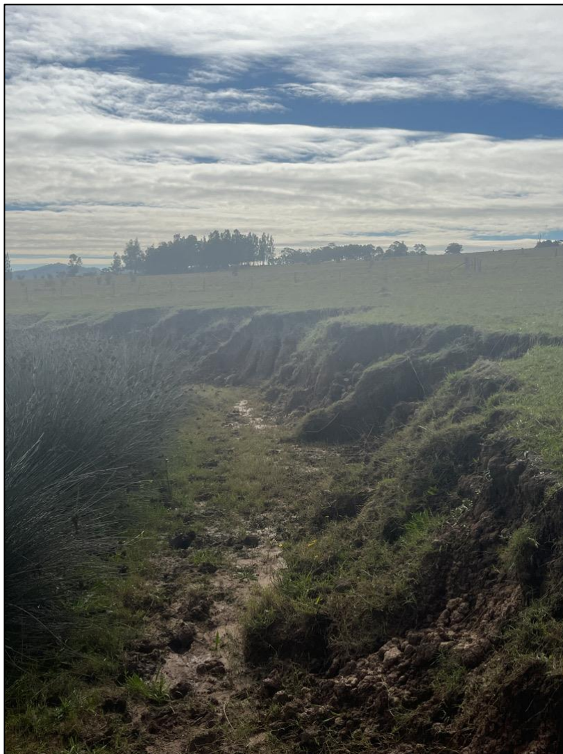
Plate 9: Bank Erosion (AEP 2024).
