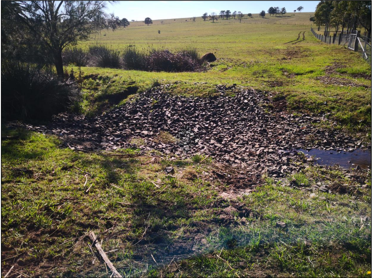
Plate 8: Crossing blocking fish passage (AEP 2024).
