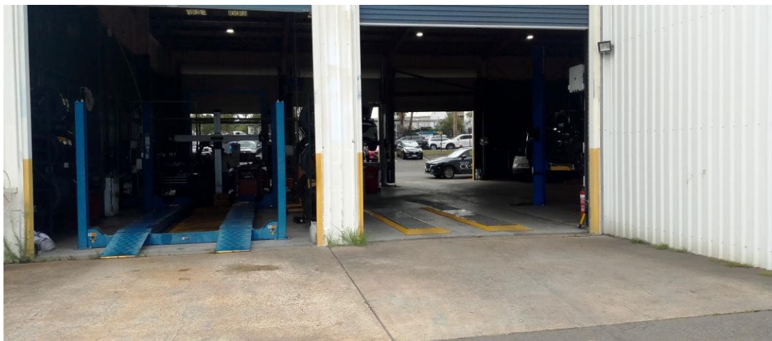
Vehicle workshop and wash bay areas
