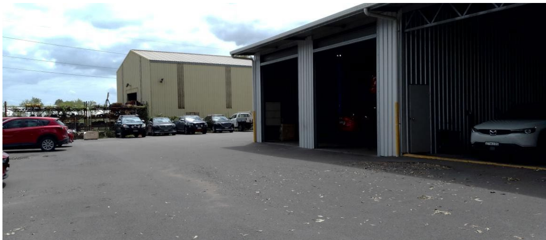
Vehicle workshop and wash bay areas
