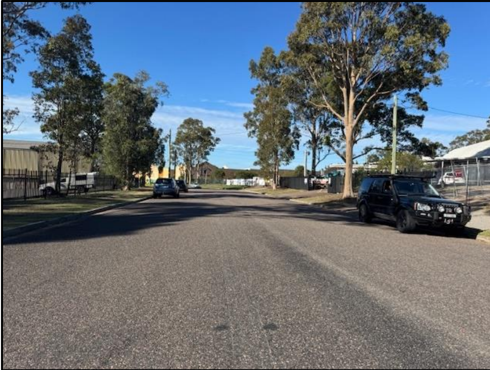
Photo 2 –Forward visibility north for driver approaching the subject site having turned into Turton Street
