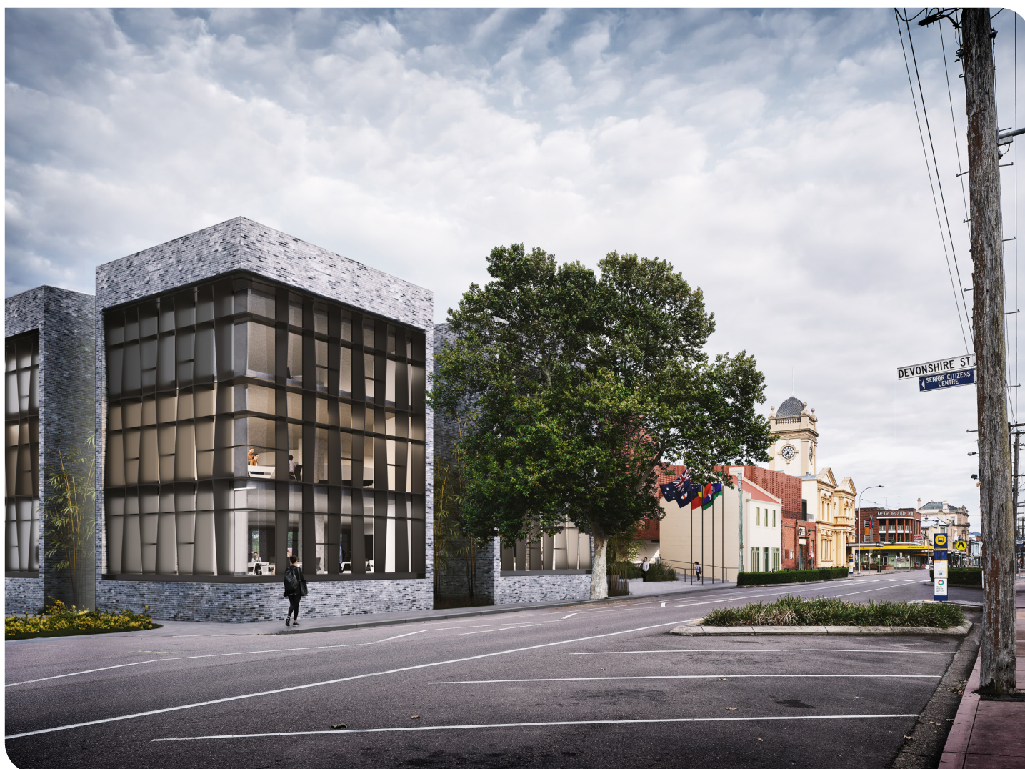
New Maitland Administration Centre, High Street, Maitland looking west
