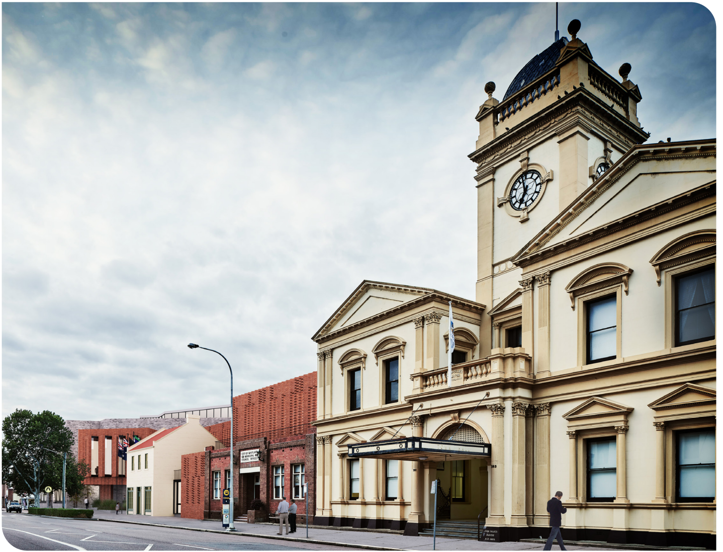
Maitland Town Hall, integrated with New Maitland Administration Centre, High Street, Maitland looking east.
