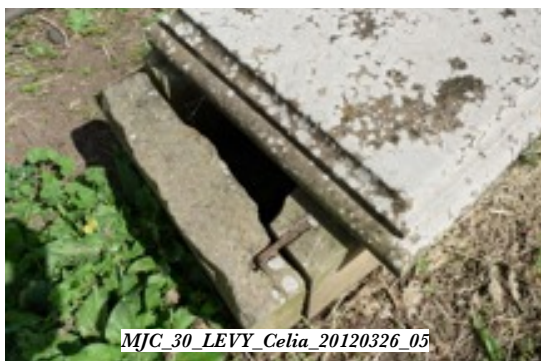
Active rusting and rust-related damage on the Celia LEVY boxtomb (#30, 1854). The photo on the right shows a corner of a side section which has fractured— probably as a function of pressure exerted with the pushing open of the top slab combined with rust jacking.
