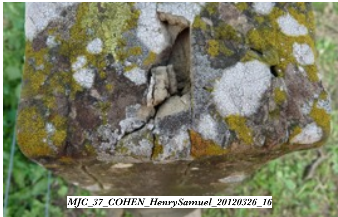
Crumbling at the top of the Henry Samuel COHEN stele (#37, 1862).
