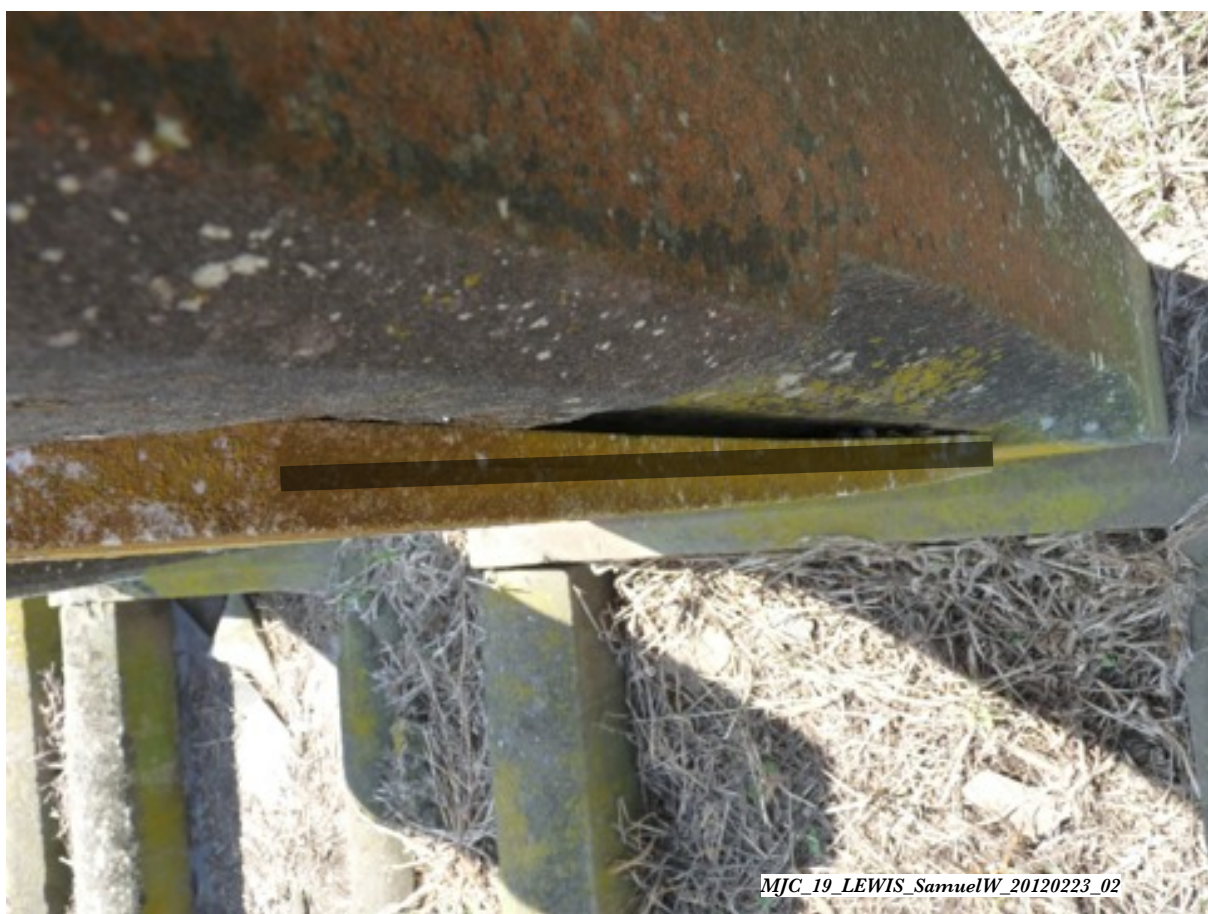
Deformation of the marble inscription panel on the Samuel W. LEWIS stele (#19, 1903, stonemason Thomas BROWNE). Opaque black line superimposed for reference and drawn over centre line of panel.
