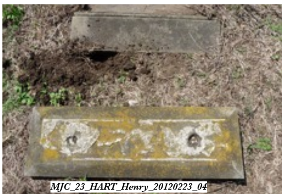
The Henry HART stele (#23, 1931) was not held securely despite cement and iron pins. At least one pin remains in the sub-base and is rusting: it will inevitably cause damage in the form of star-cracking and, subsequently, the fracturing of the stone.
