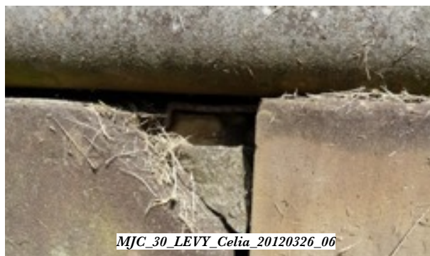
Active rusting and rust-related damage on the Celia LEVY boxtomb (#30, 1854). The photo on the right shows a corner of a side section which has fractured— probably as a function of pressure exerted with the pushing open of the top slab combined with rust jacking.
