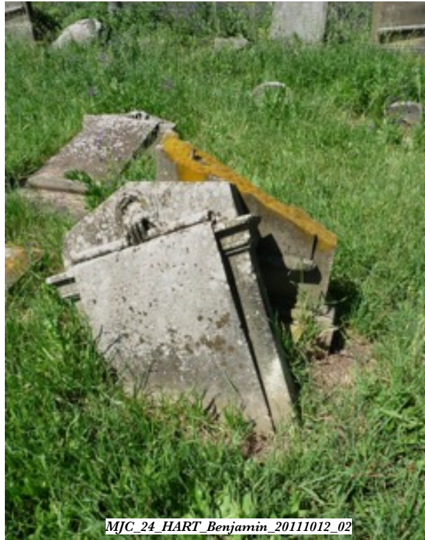
The Benjamin HART stele (#24, 1905) is at considerable risk of ongoing impact damage: as clearly shown by heavy chipping, scratching, and cuts which occurred from lawn mowers during the site survey.
