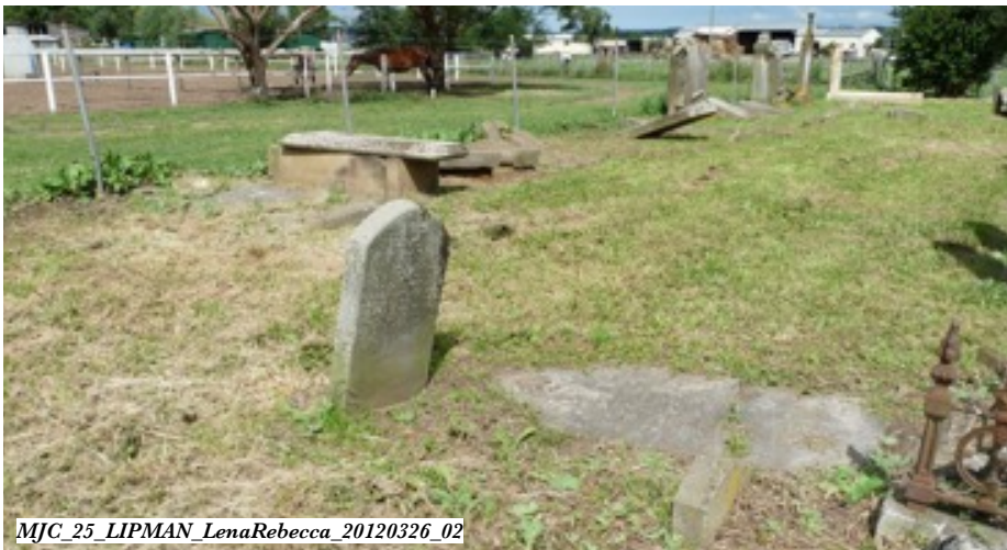
Foreground monuments for Lena Rebecca LIPMAN (#25, 1882, on left) and George Judah COHEN (#14, 1889, on right) are both High Conservation Priorities: the former as it has a structural lean, the latter being at risk of accelerated deterioration as well as further impact damage lying on the ground.
