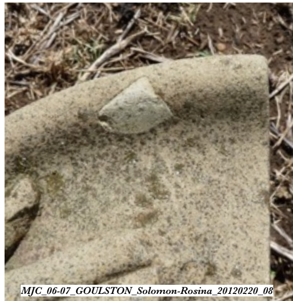
Plastic repair in the Ravensfield Sandstone of the Solomon GOULSTON stele (#6, 1862).
