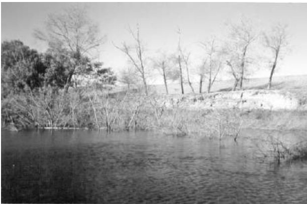
An example of streambank erosion along the Hunter River. Extensive land clearing along streambanks has made this a common sight.
