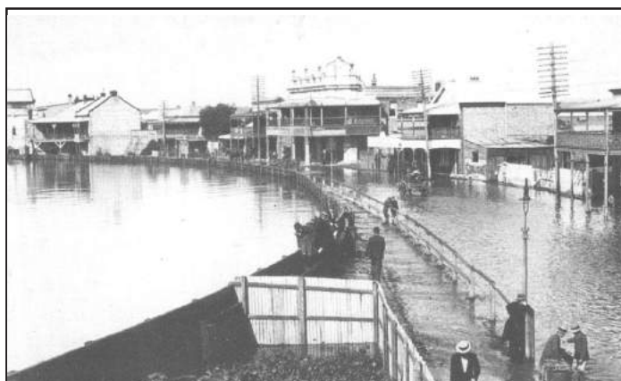
Flooding in eastern High Street, West Maitland. A timber wall had been constructed to keep the river out of High Street. This was the original course of the river until the change in 1893. This photograph could have been taken then or possibly during the 1913 flood.
