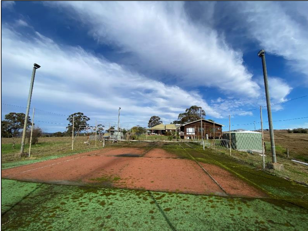
Plate 5: Looking south over the modified western portion of the site (built up tennis court area).
