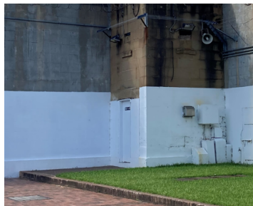
Figure 2 | Tower 1 – Ground Level
