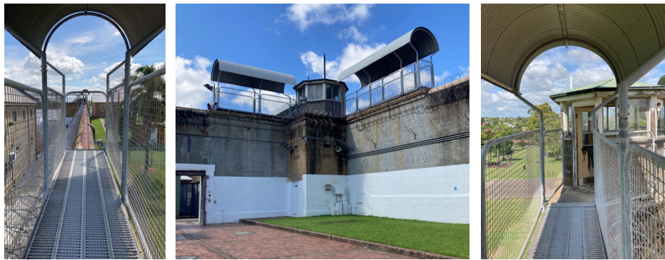
Figure 1 | Maitland Gaol Tower + Gantries
