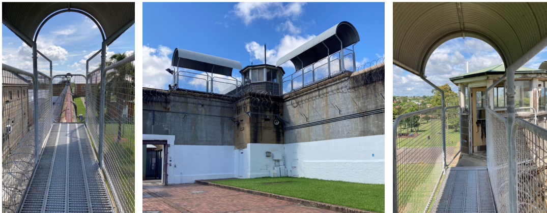
Figure 1 | Maitland Gaol Tower + Gantries
