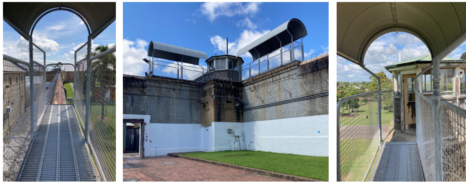
Figure 1 | Maitland Gaol Tower 1 + Gantries
