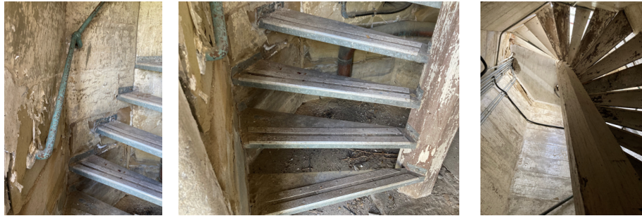
Figure 3 | Tower 6 – Existing Stair Access
