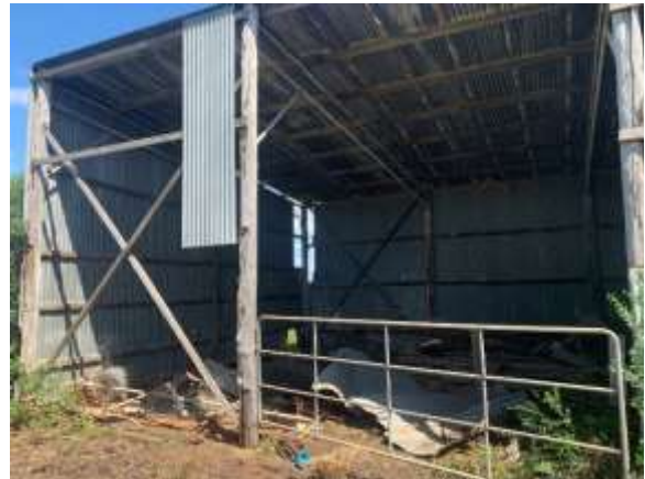
Farm shed – NE portion of site (former Lot 32)
