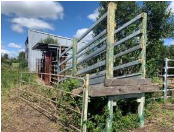
Cattle Ramp – NE portion of the site (former Lot 32)
