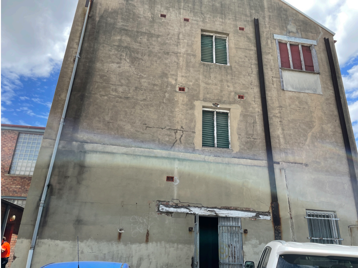
Figure 3 – External View of the Existing Building (Eastern Elevation)
