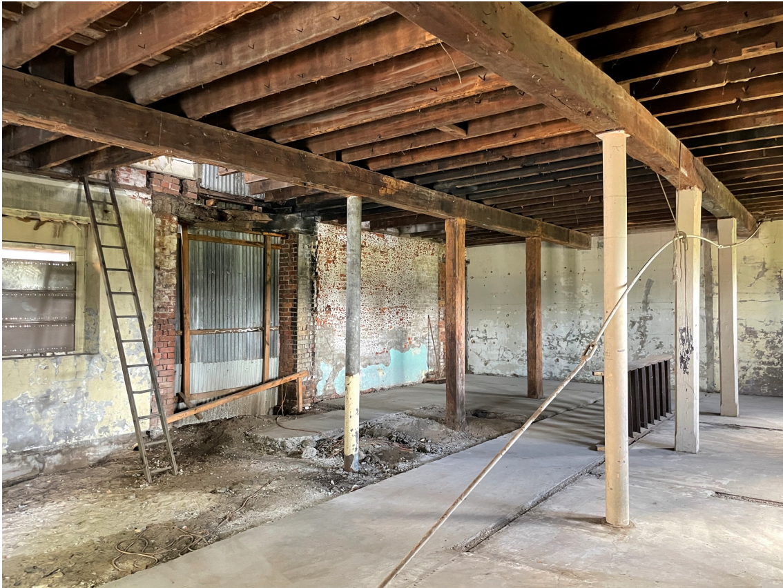
Figure 5 – Internal View of the Existing Building (Looking South West)
