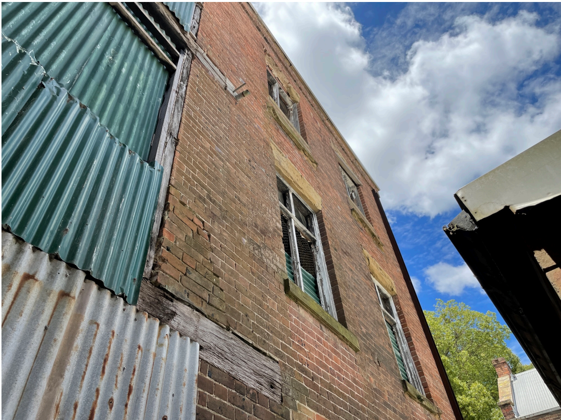
Figure 4 – External View of the Existing Building (Southern Elevation)
