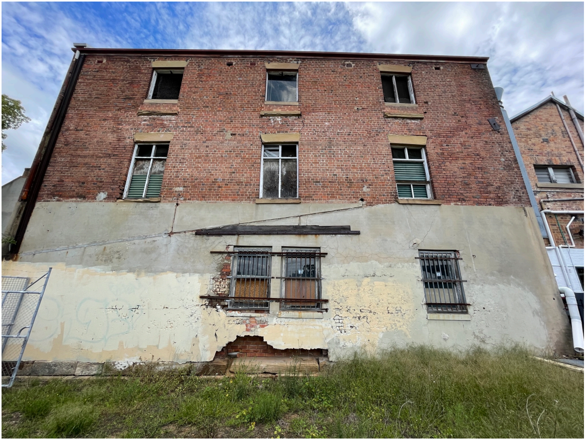
Figure 2 – External View of the Existing Building (Northern Elevation)
