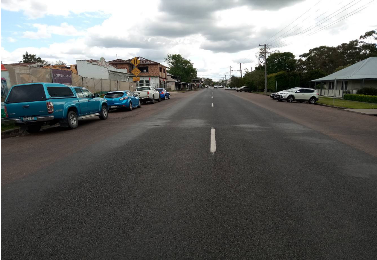
Photograph 5 – Swan Street adjacent to the site
