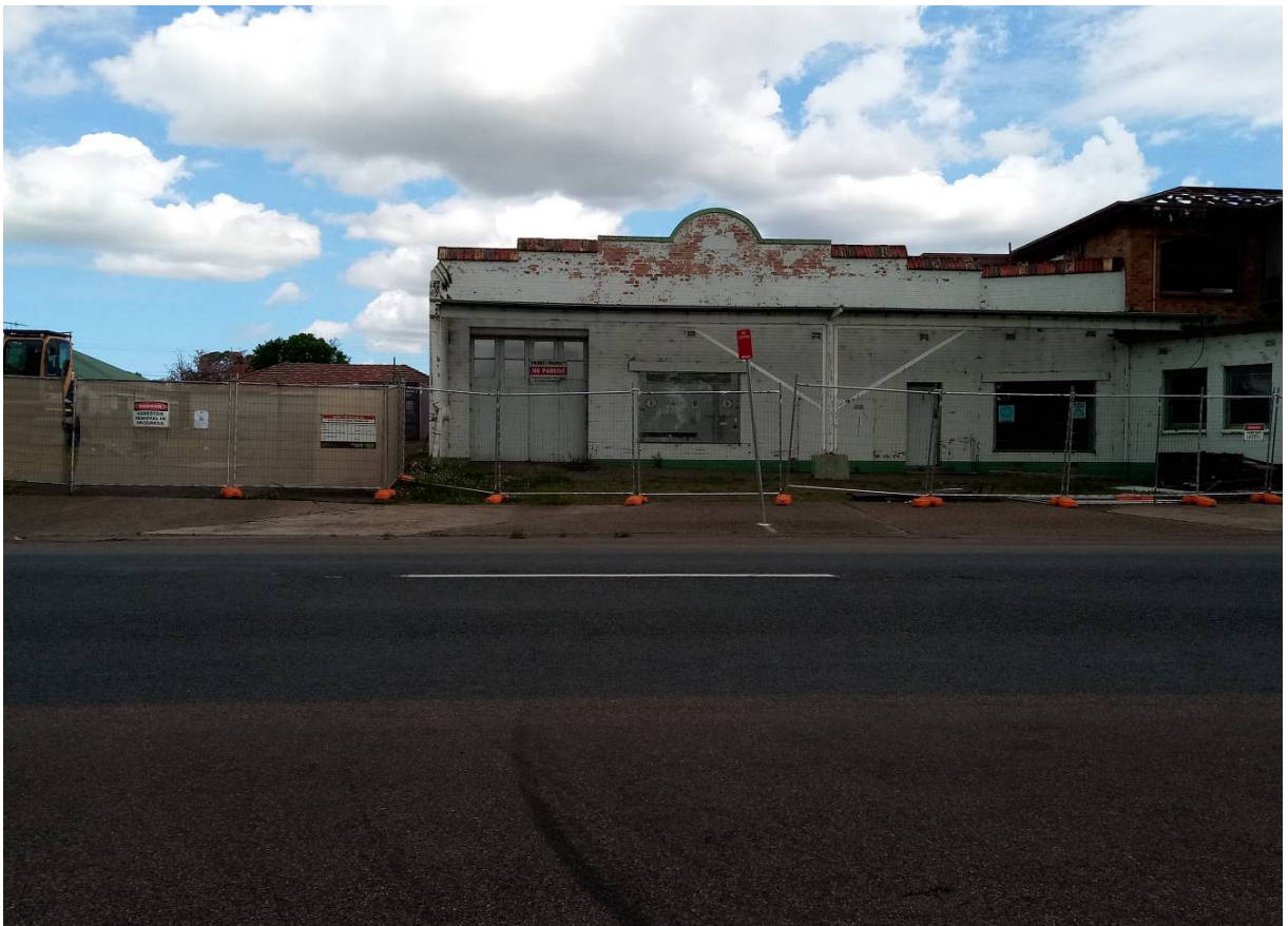
Photograph 3 – Wide access crossing at Swan Street servicing 3 lots of the existing site
