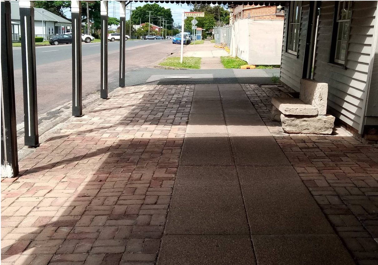
Photograph 10 – Swan Street footpath near Market Street, fronting and west of the site
