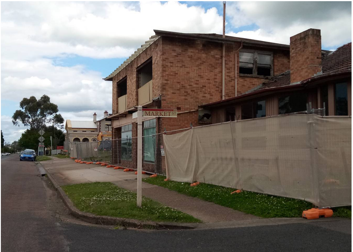
Photograph 1 – Existing site at Swan Street
