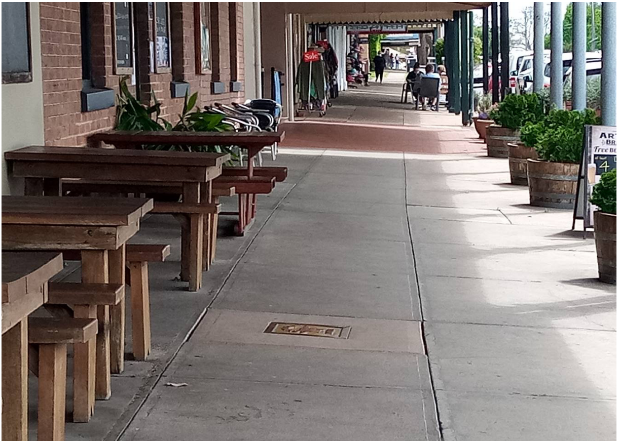
Photograph 11 – Full width footpath Swan Street west of Northumberland Street
