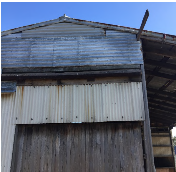
Photograph 15: Showing ACM panels within the building on site
