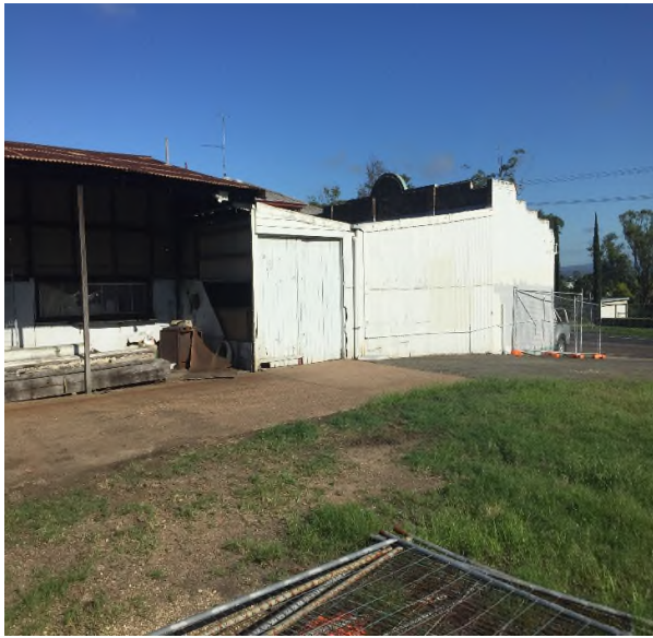
Photograph 13: Looking at building in western portion of site
