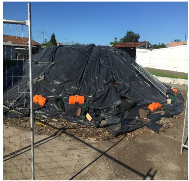
Photograph 6: Closeup of stockpile showing mulch bunding around base and black plastic covering
