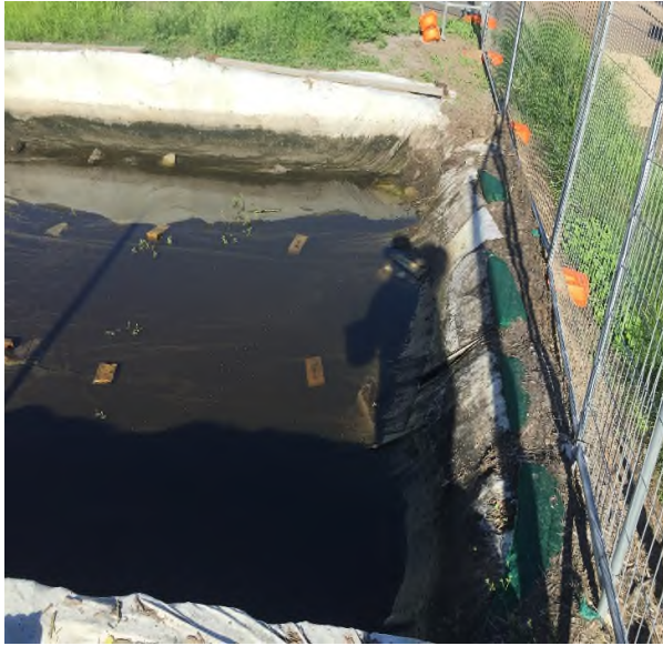
Photograph 9: Showing silt barrier at northern end of sediment basin
