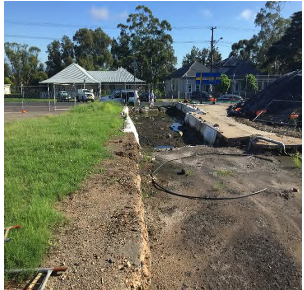
Photograph 12: Looking north at sediment basin and cut area
