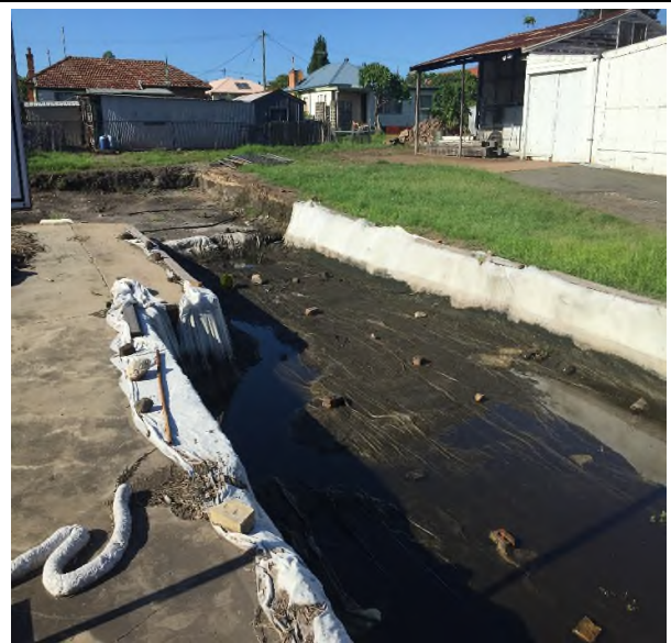
Photograph 8: Sediment basin on northern border of site, looking south
