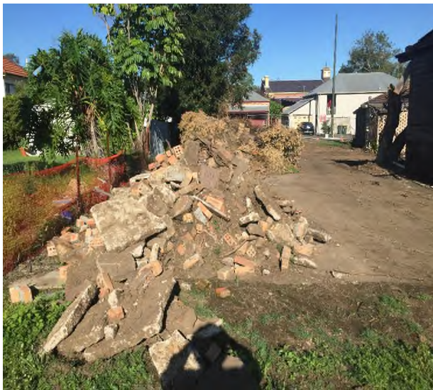
Photograph 4: Construction material stockpiled on southern boundary of site, looking west
