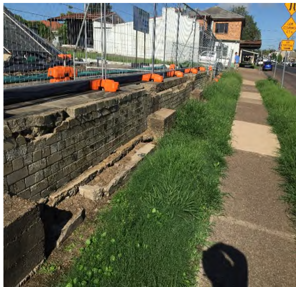
Photograph 19: Showing brick and concrete building footing
