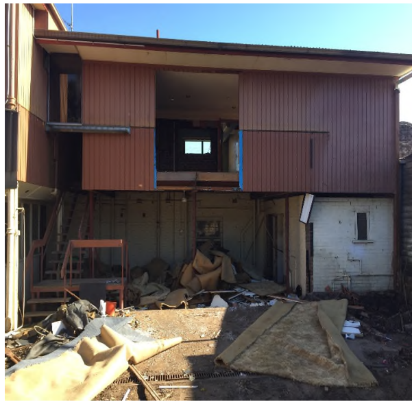
Photograph 17: Showing rear of 2-storey building, looking north
