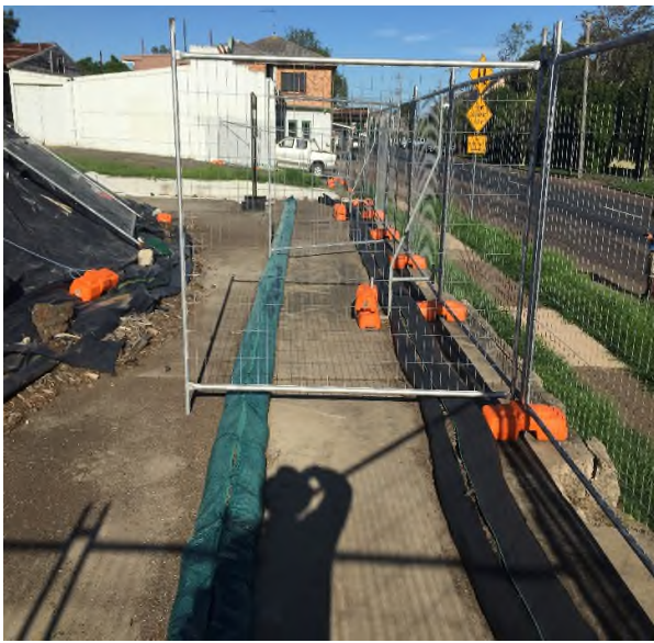
Photograph 5: Silt barriers on the northern side of the stockpile
