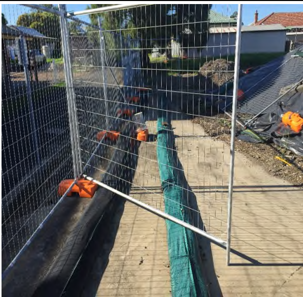
Photograph 7: Silt barriers on the eastern side of the stockpile, looking south
