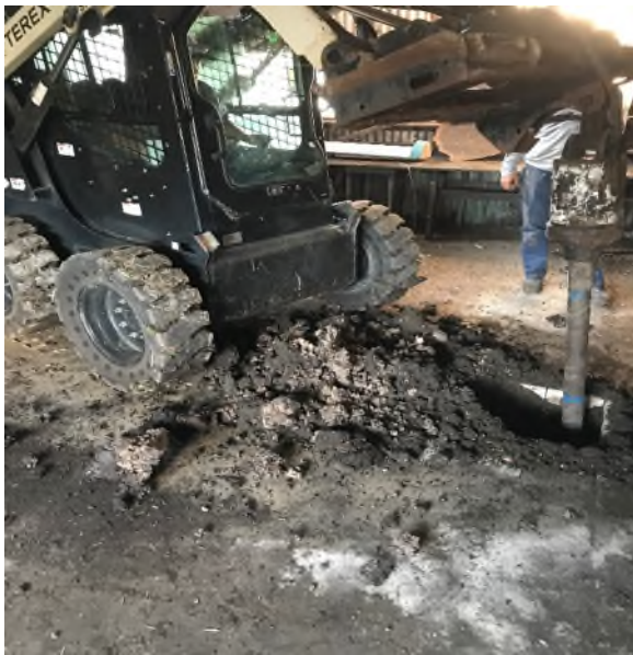
Photograph 27: Showing borehole location BH18 within the existing shed
