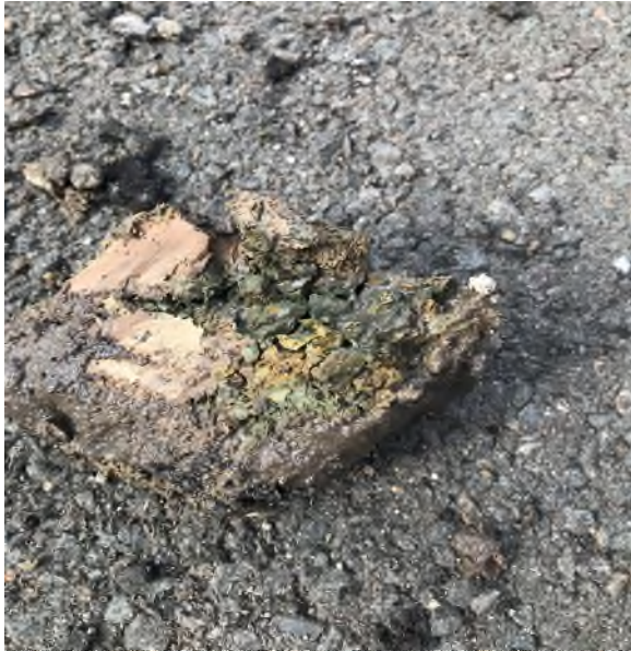
Photograph 25: Showing material from BH14 with green staining on clay layer (1.4 – 2.1mbgs)
