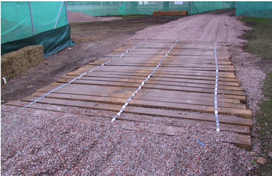
Figure 10 – Example of acceptable Tree Protection Area ground protection
