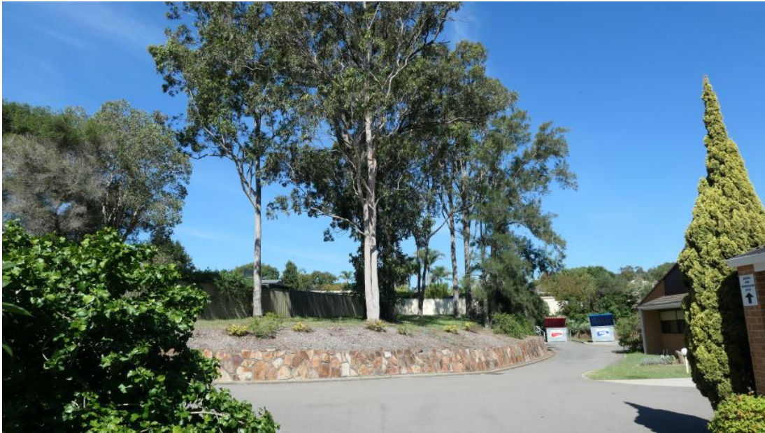
Figure 8 – Group 3 is a significant stand of endemic trees and these have been a focus of tree retention on the project. It is proposed to retain existing ground levels around the trees and a new retaining wall will be built in front of the existing level change in order to protect and retain the trees (Photo: Arterra 15/4/2020)
