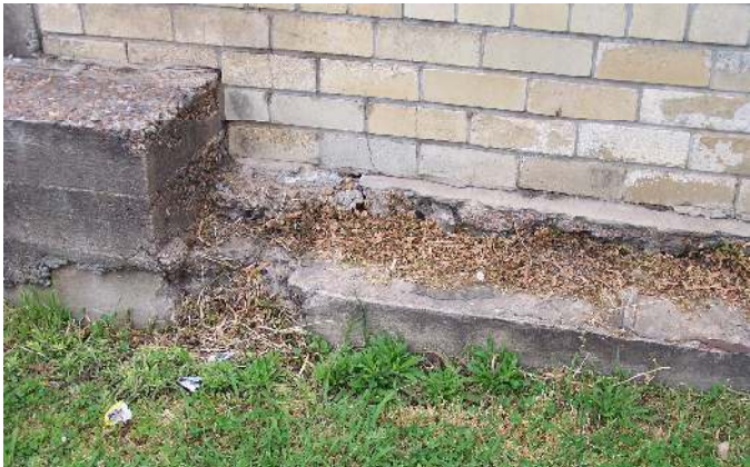
Figure 2.20 [left] Showing an exemplary sector of retaining wall, close to the Swan/William Streets corner: In this sector, the remains of verandah footing and floor can be seen protruding below brickwork. The upper surface exposed at this level was the edge of a concrete floor of a workshop constructed in connection with the Volvo truck franchise of Griffin Motors –probably the reason for introduction of fill. Paul Rheinberger Scale: 200mm
