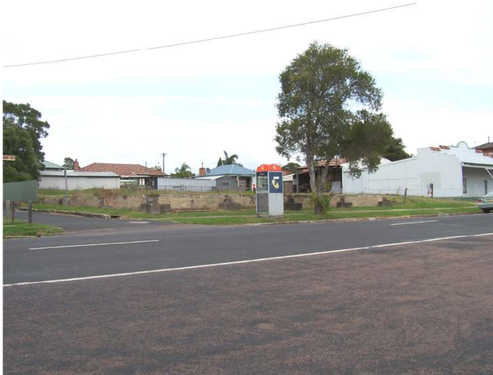
Figure 2.19 Here can be seen the full extent of the brick retaining wall, from left to right commencing at the termination of a metal fence on the western side of William Street and running north to the Swan Street corner, then running west with five concrete buttresses to the point at which the surface declines to road level Paul Rheinberger No Scale
