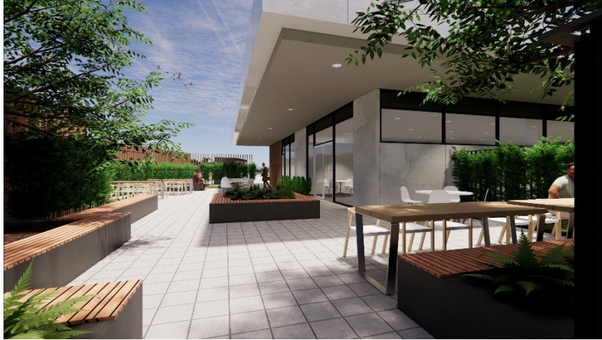
Figure 2: a view towards the staff outdoor area, which is dedicated to worker amenity and the safe and secure pedestrian movement of staff.
