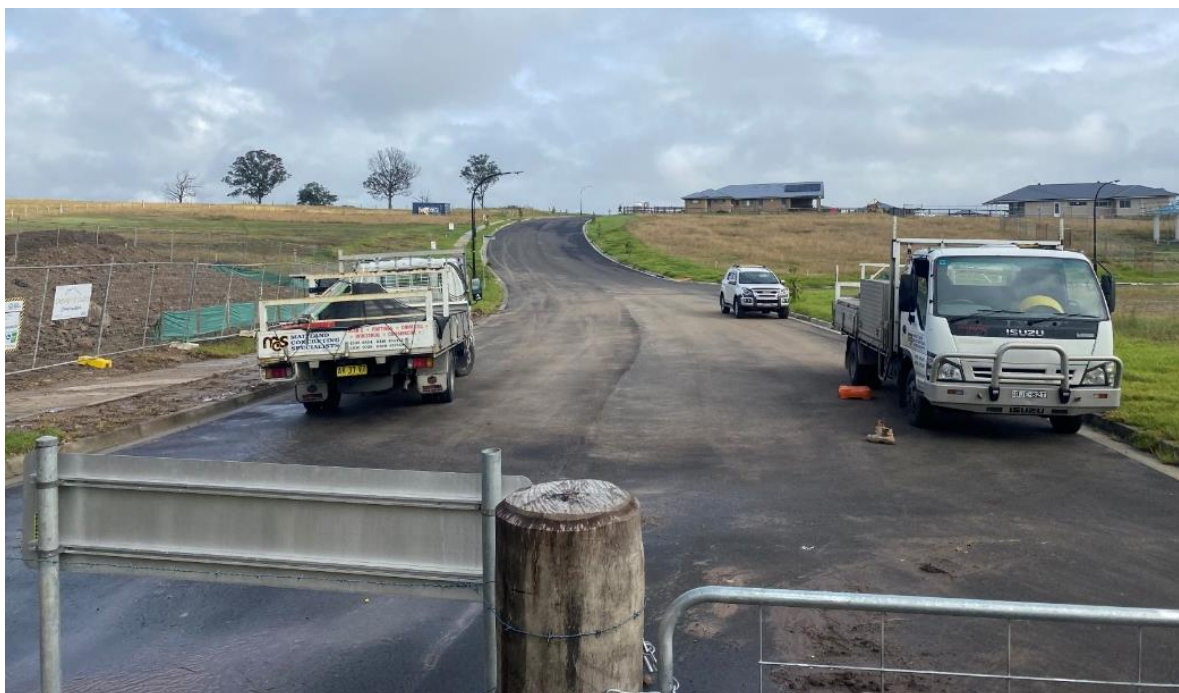
Plate 10: Collaroy Road constructed west
