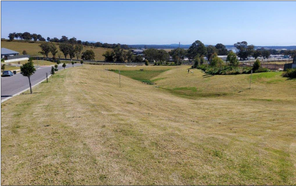
Plate 17: T17 Stormwater device east of site is managed and used as open space
